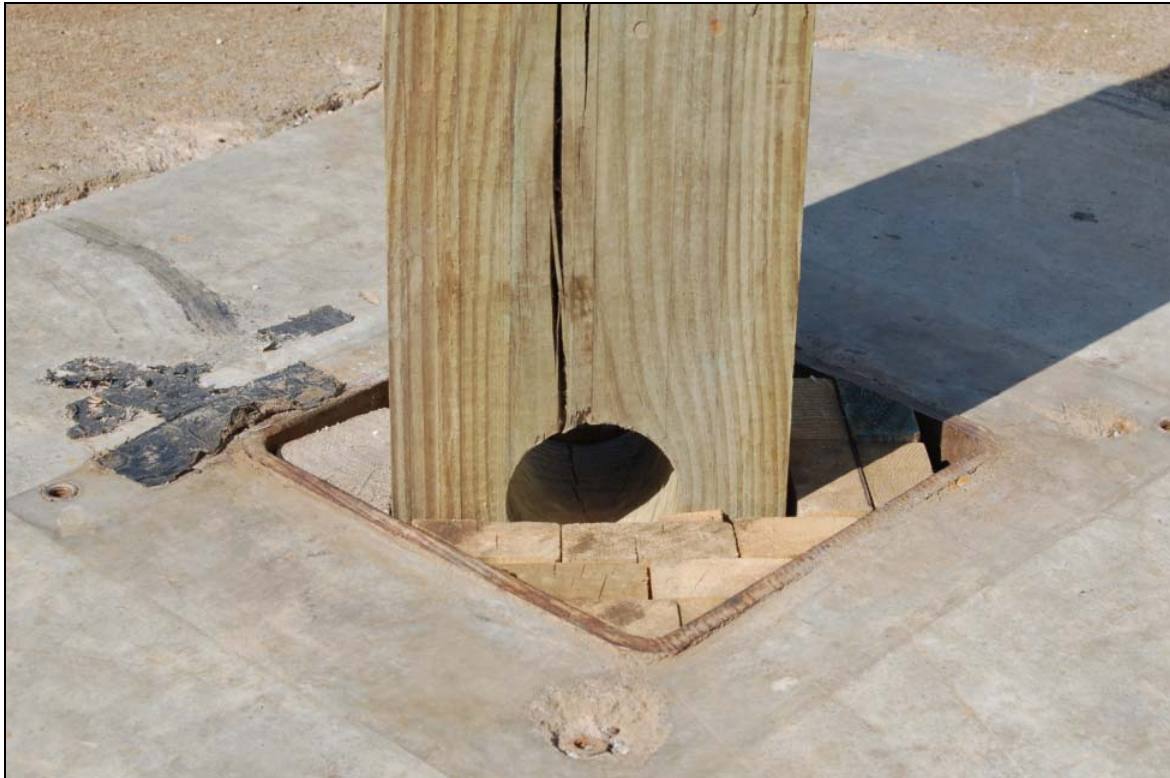
Figure 3. Shimmed CRT in Rigid Sleeve
