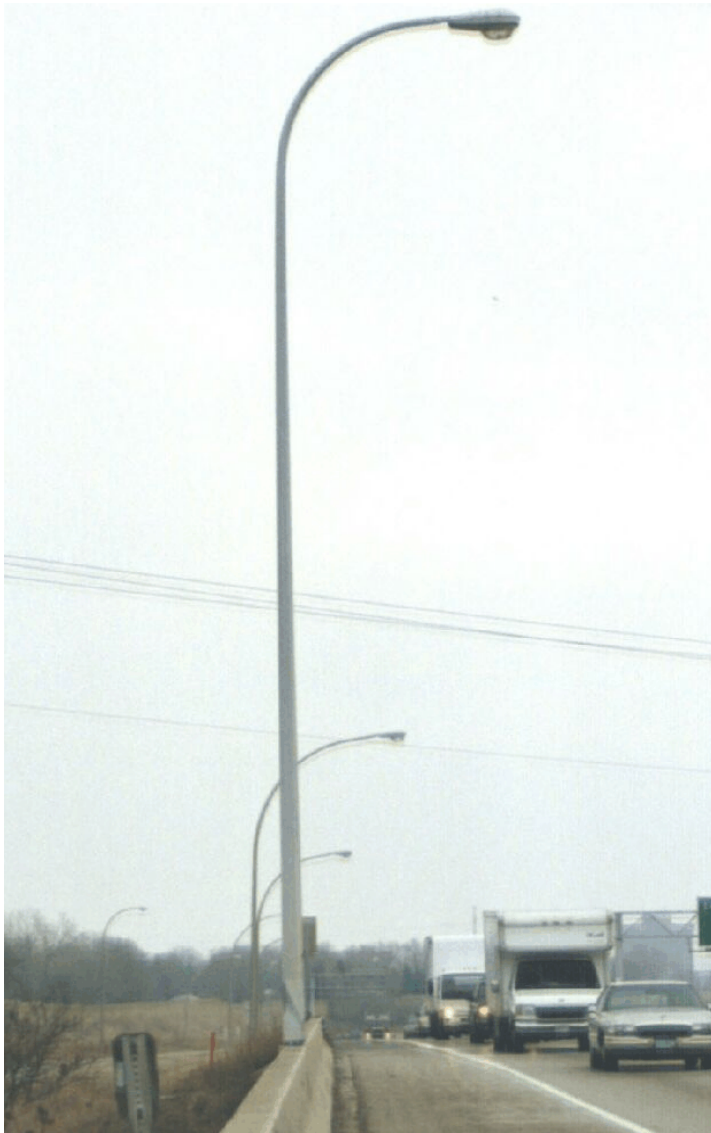
Figure 9. Luminaire Supports Mounted on Top of the Traffic Barrier
