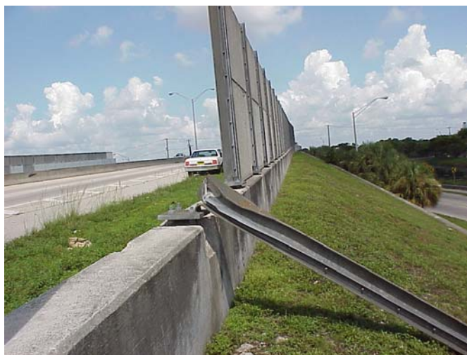
Figure 18. Failure of a Smooth Continuous Attachment
