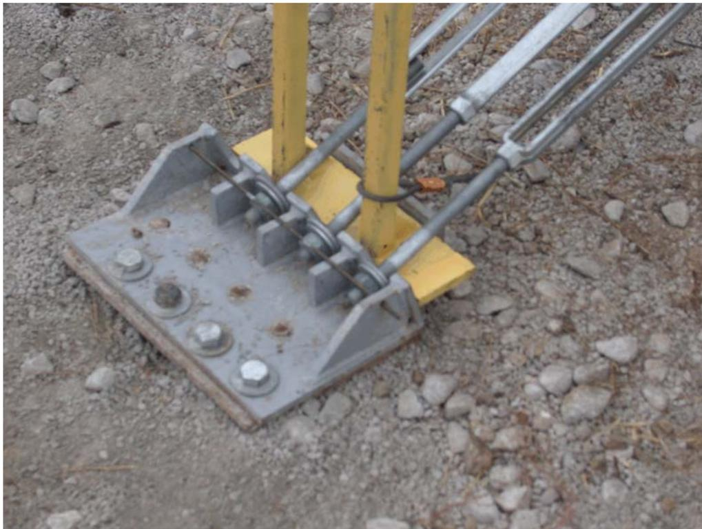
Figure 65. Cable to Keep Cable Release Lever Attached to System, Design No. 2
