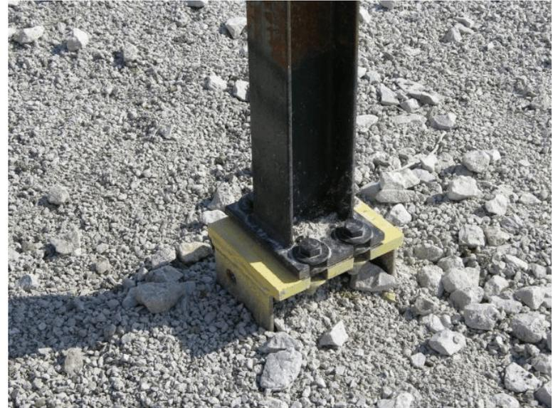
Figure 93. End Terminal Line Post Details, Design No. 3
