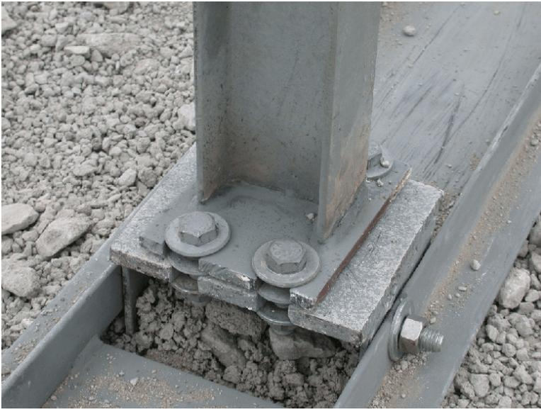
Figure 23. Slip-Base Post Details, Design No. 1
