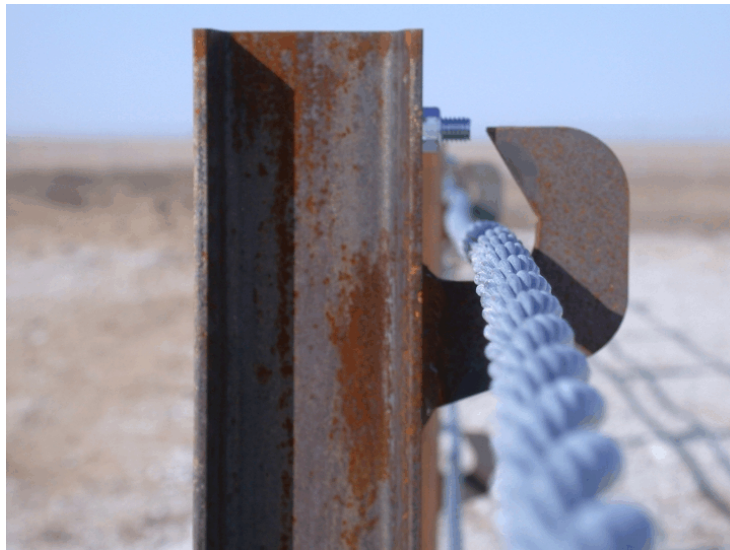
Figure 79. Line Post Nos. 26 through 45 Cable Brackets, Design No. 3
