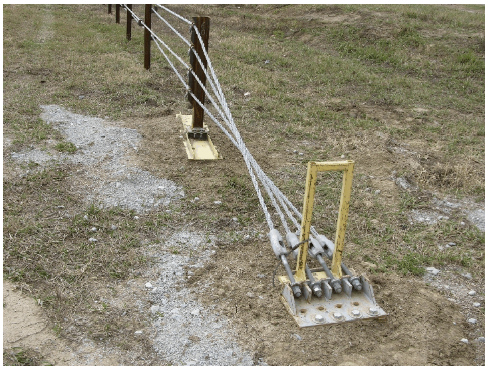
Figure 56. Low-Tension Cable Median Barrier, Design No. 2
