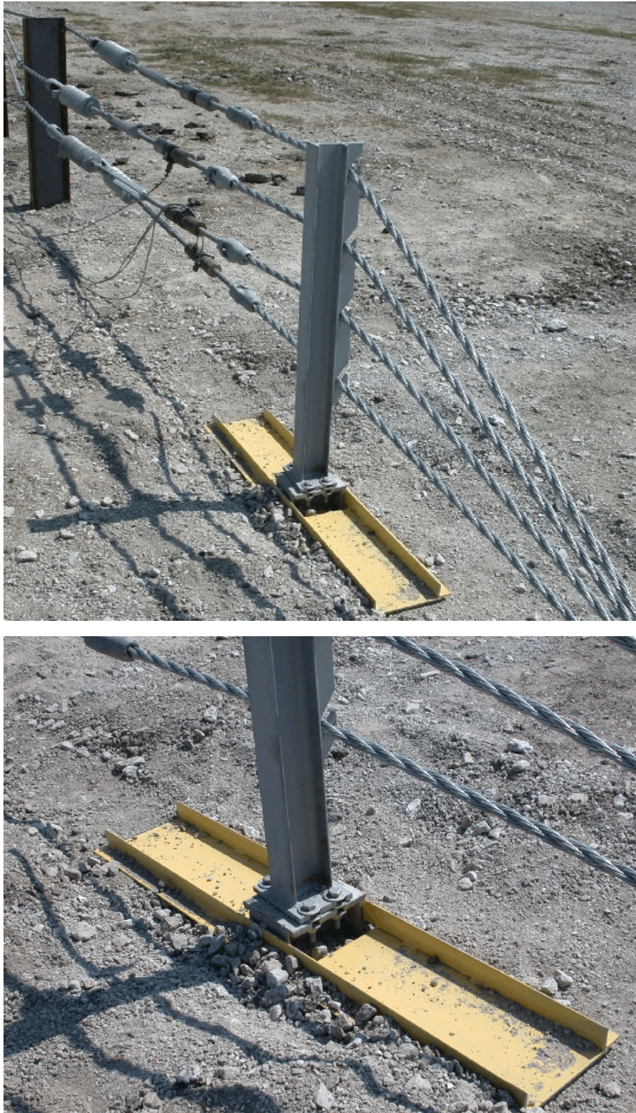
Figure 32. Cable Support Post, Design No. 1
