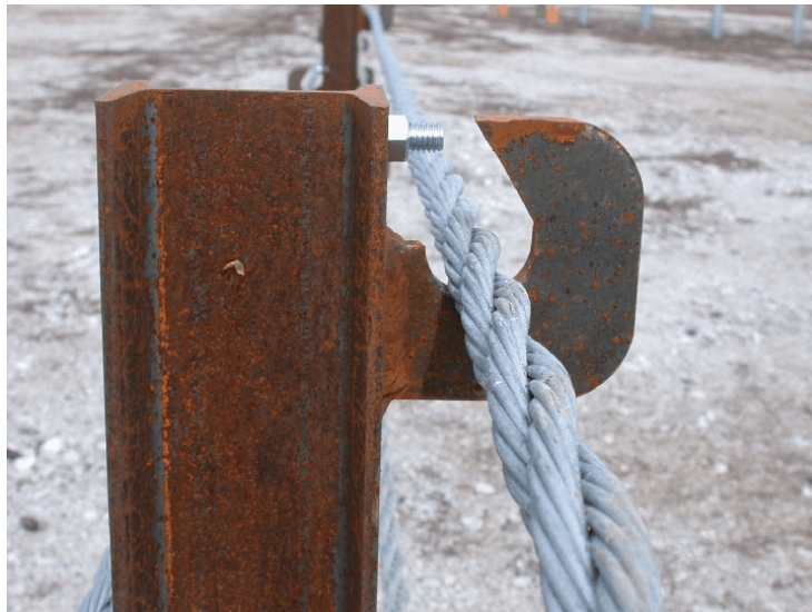
Figure 80. Line Post Nos. 3 through 25 and 46 through 59 Cable Brackets, Design No. 3
