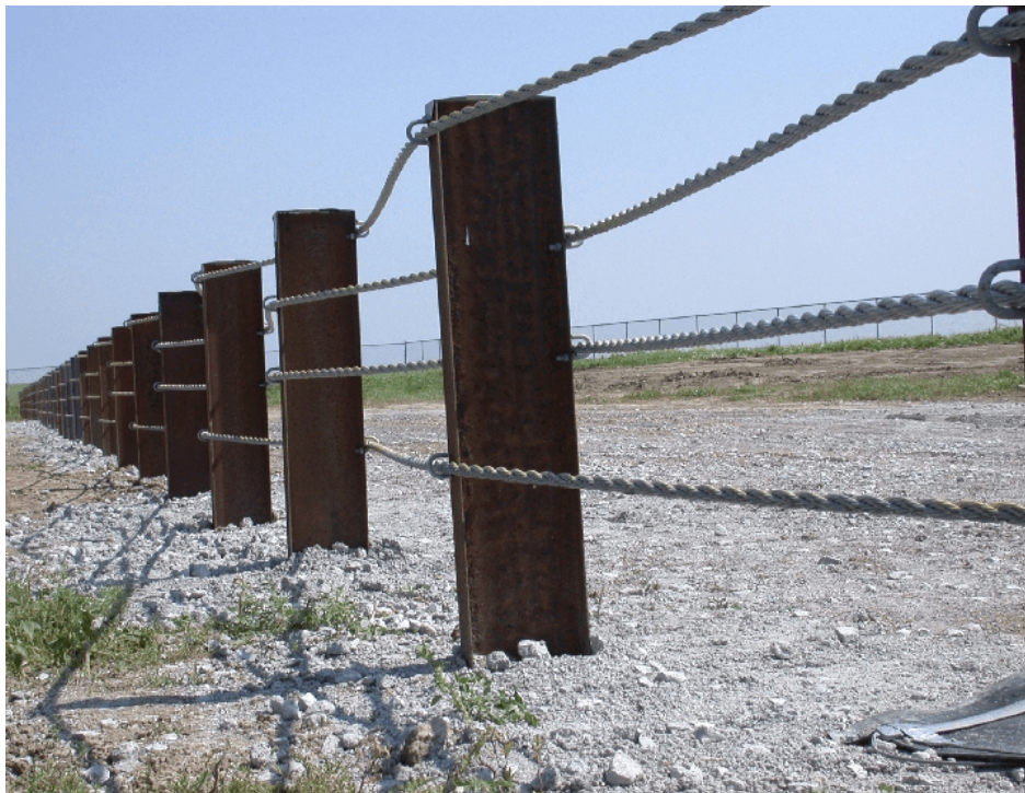
Figure 30. Low-Tension Cable Median Barrier, Design No. 1
