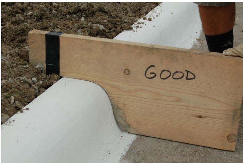
Figure 16. 152-mm (6-in.) AASHTO Type B Curb Construction and Test Layout 29
