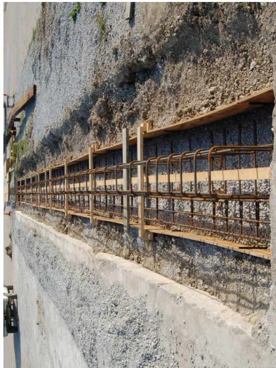
Figure 31. Aggregate Base and Foundation Slab Formwork and Steel Reinforcement
