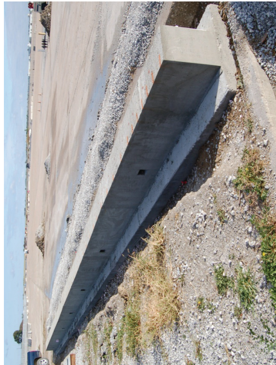
Figure 33. Inner Concrete Core Wall
