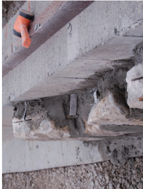
Figure 35. Anchorage for Rough Stone Masonry Facade
