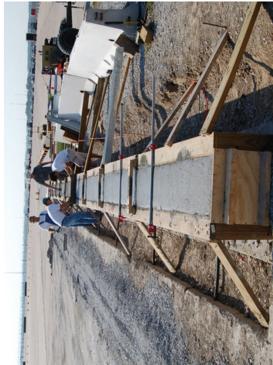
Figure 32. Cast-In-Place Construction for Inner Concrete Core Wall
