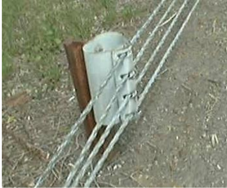
Figure 11. Steel-Post 4-Cable Guardrail System Installed In Field [15]
