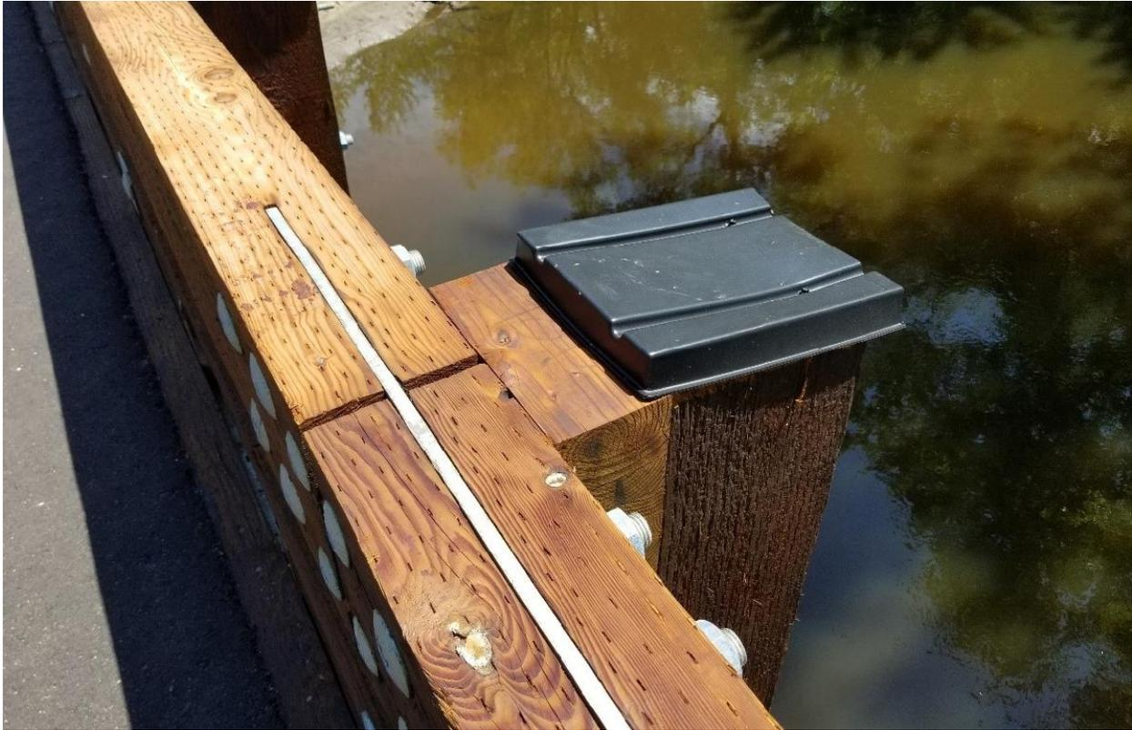
Figure 60. Plastic Cap Covering Top of Post [83]
