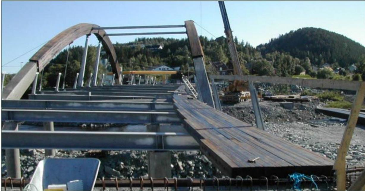
Figure 47. Stress-Laminated Deck Built on Steel Cross-Beams [73]
