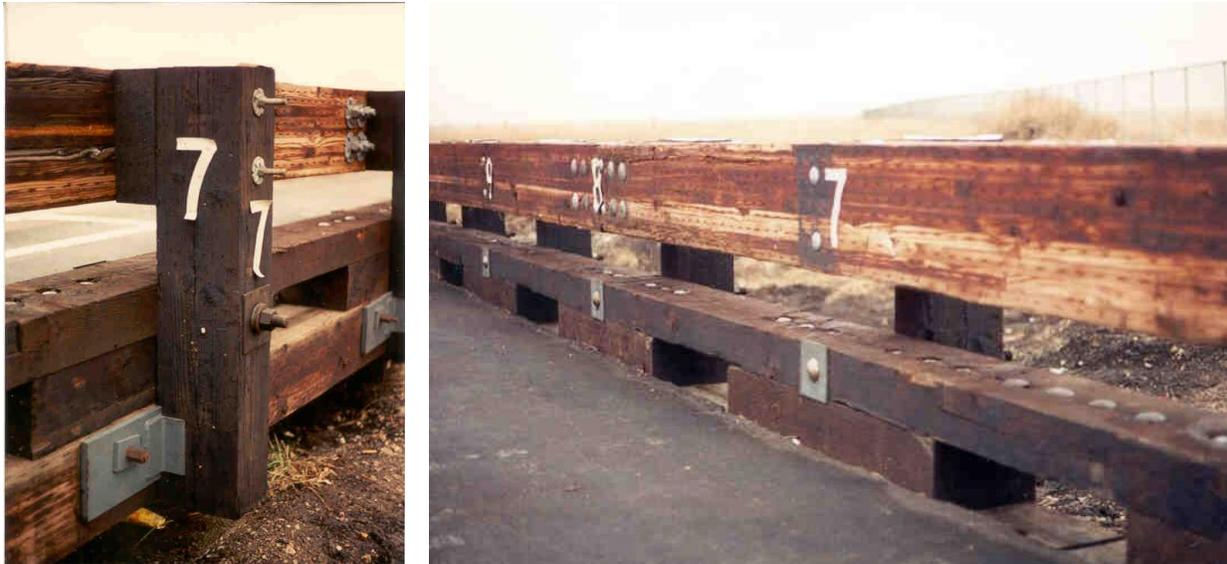
Figure 2. GC-8000 Timber Bridge Railing on Longitudinal Glulam Deck [16]
