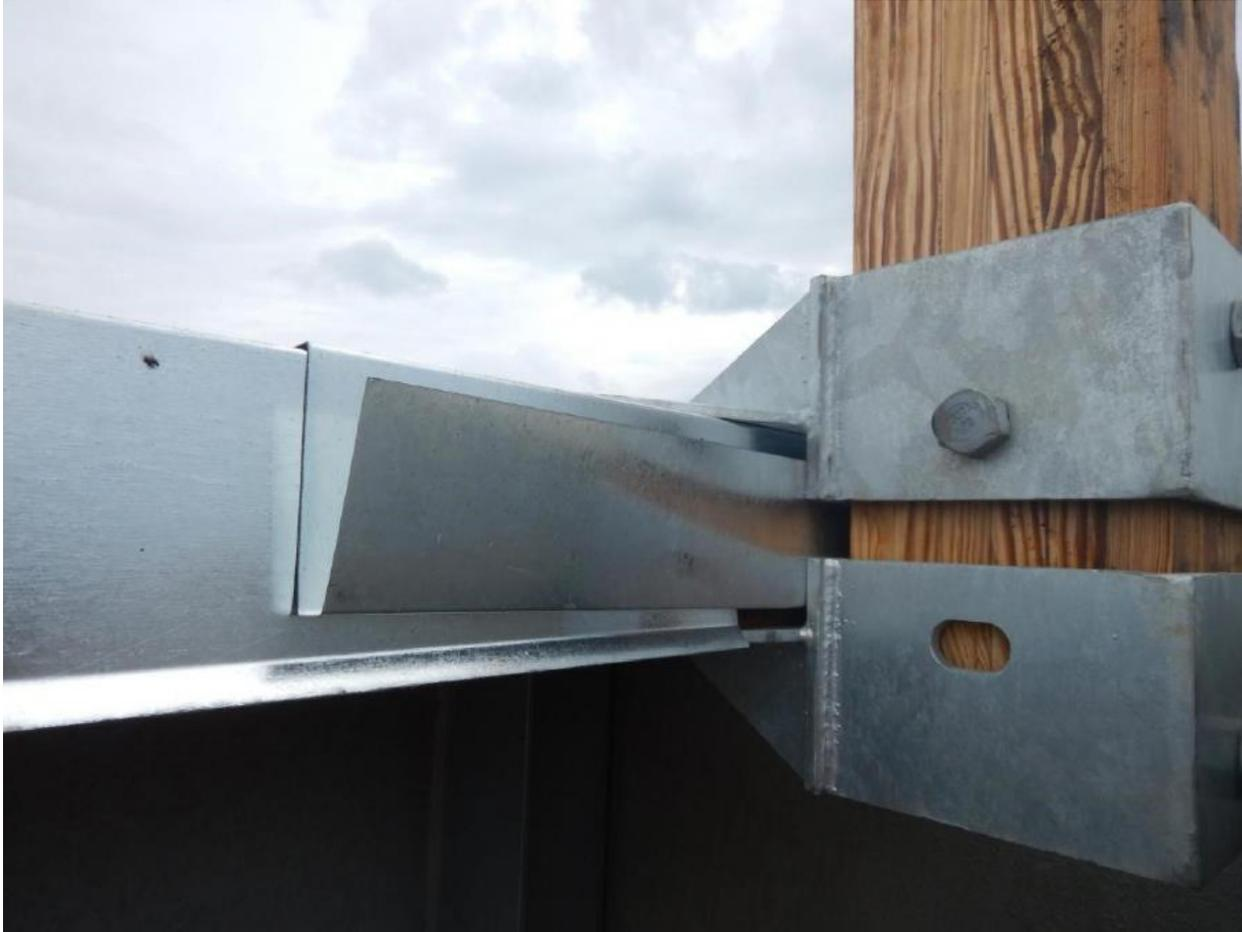
Figure 58. Flashing on Transverse Timber Bridge Deck Edges, Covering Panel End Grain [83]
