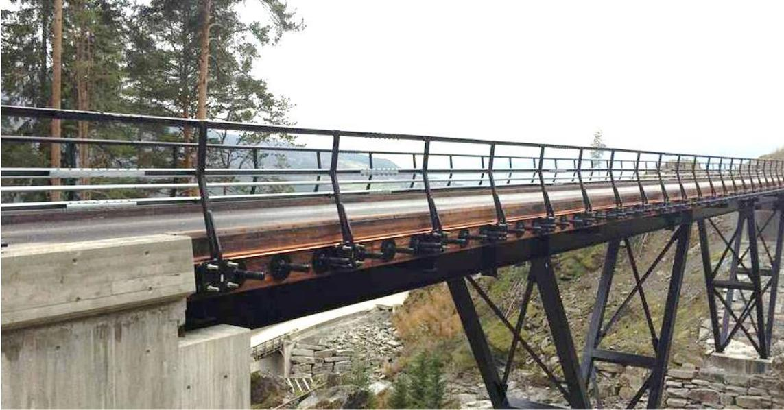
Figure 11. Timber Bridge Railing for Stress-Laminated Deck Built by AB Varmförzinkning [30]
