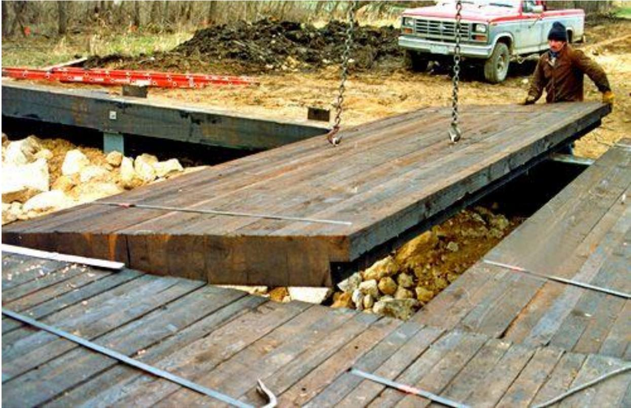
Figure 44. Assembly of Spike-Laminated Deck Panels into Bridge Deck [63]
