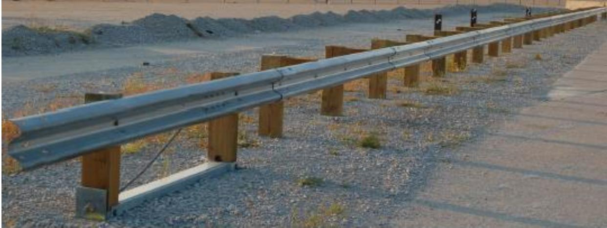
Figure 29. MGS Utilizing SYP Grade No. 1 Posts [43]
