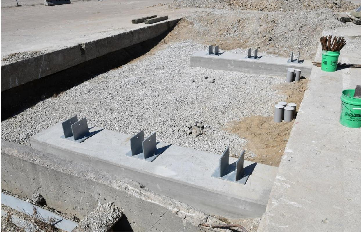
Figure 172. Fully Cast Substructure and Steel Bearing Assemblies, Test No. TRTD-1
