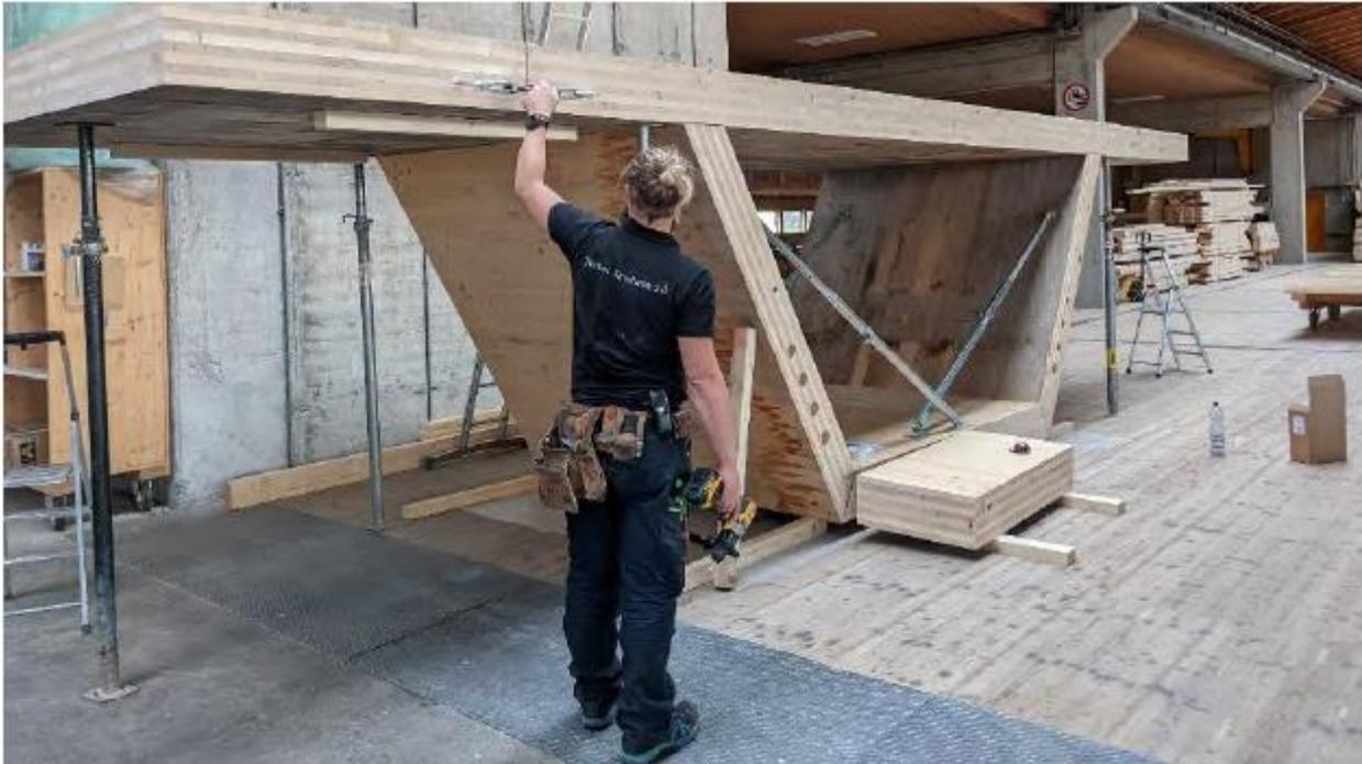
Figure 50. Timber Glulam Box Girder [78]
