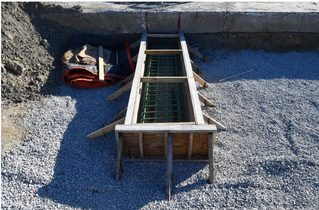
Figure 171. Forms for Substructure with Rebar Cage, Test No. TRTD-1
