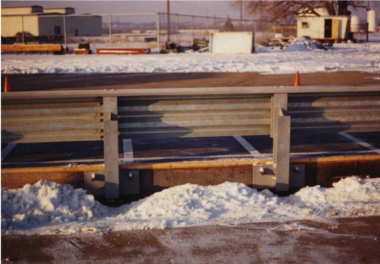
Figure 5. TBC-8000 Steel Bridge Railing on Longitudinal Timber Bridge Deck [19]
