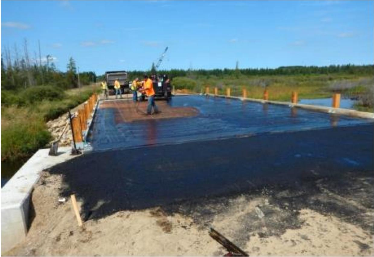
Figure 54. Tack Coat Applied to Timber Bridge Demonstration Bridge in Minnesota [83]
