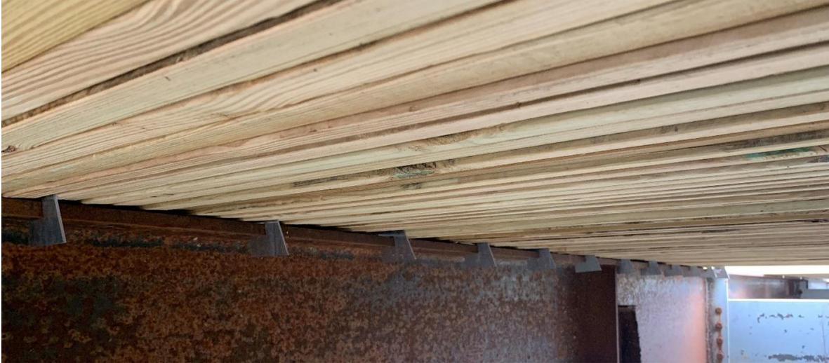
Figure 37. Uneven Bearing of Nail-Laminated Decks on Supports [7]
