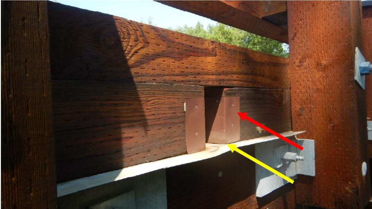
Figure 59. Flashing on Longitudinal Timber Bridge Deck Panels and Railing Scuppers. Top arrow: points to the flashing protecting the ends of the bridge scuppers. Bottom arrow: points to the flashing which carries water away from the bridge deck [83]
