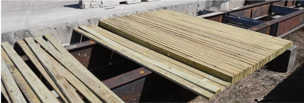
Figure 34. Transverse Nail-Laminated Deck Construction [7]
