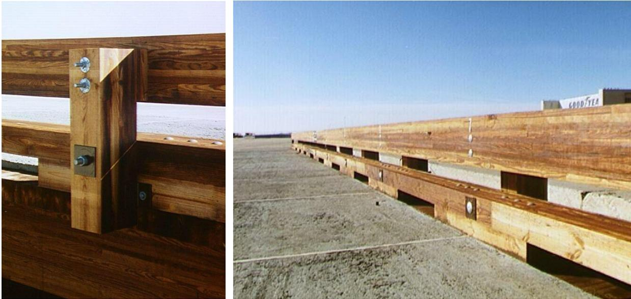
Figure 6. NCHRP 350 TL-4 Glulam Timber Bridge Railing with Curb on Transverse Glulam Deck [25]
