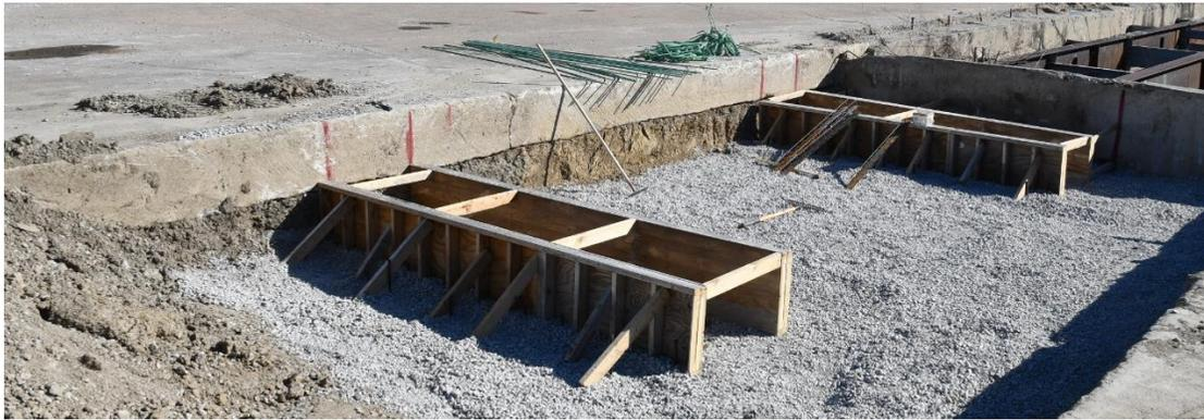
Figure 170. Forms for Test No. TRTD-1 Substructure, Test No. TRTD-1
