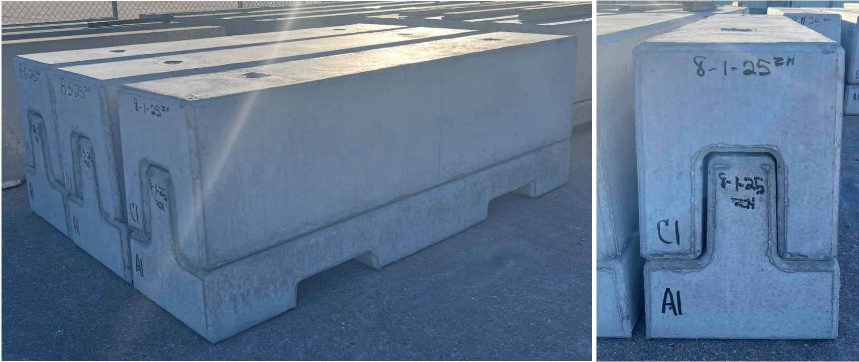
Figure 82. Staggered, Interlocking PCB Prototype Photographs
