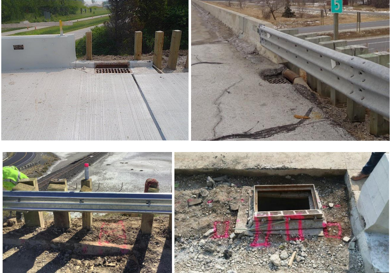
Figure 3. Photographs of Actual AGT Installations with Obstructed AGT Posts
