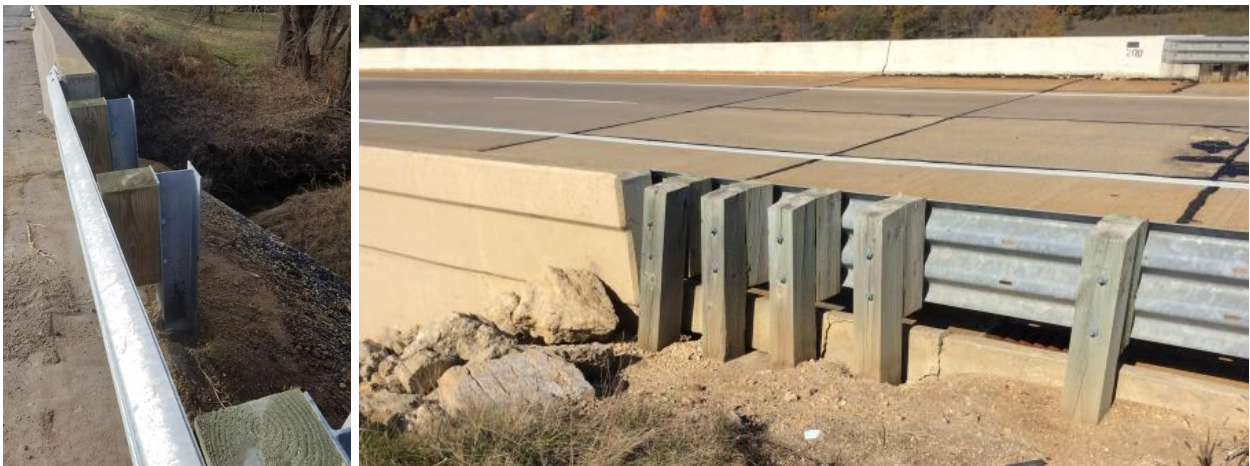
Figure 4. Photographs of AGTs Installed on Slopes
