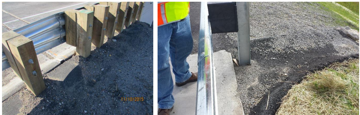
Figure 5. Photographs of AGT Posts Within Asphalt or Concrete Pavements
