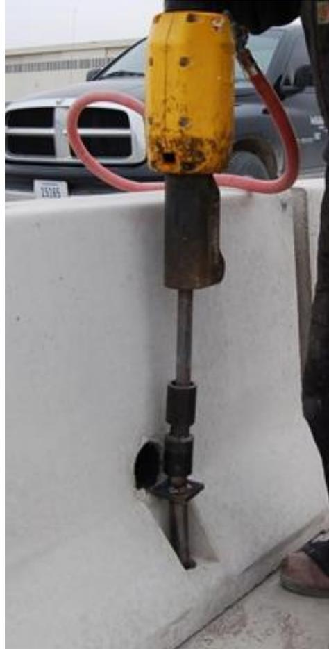
Figure 1. Asphalt Pin Tie-Down for F-Shape PCBs
