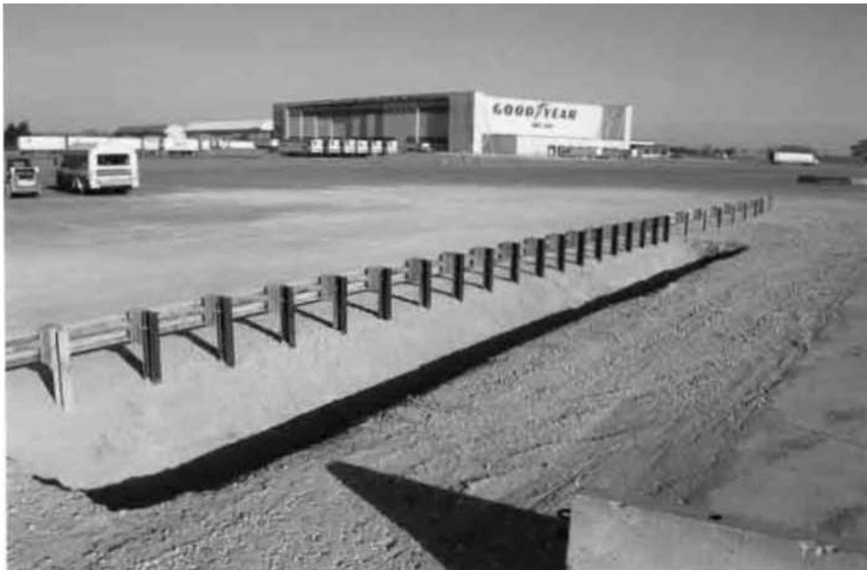
Figure 1. W-beam Guardrail Adjacent to a 2:1 Foreslope, Test No. MOSW-1 [2]
