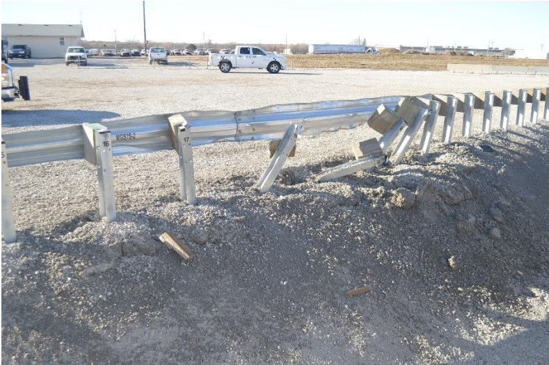
Figure 52. System Damage, Test No. MGS7S-2
