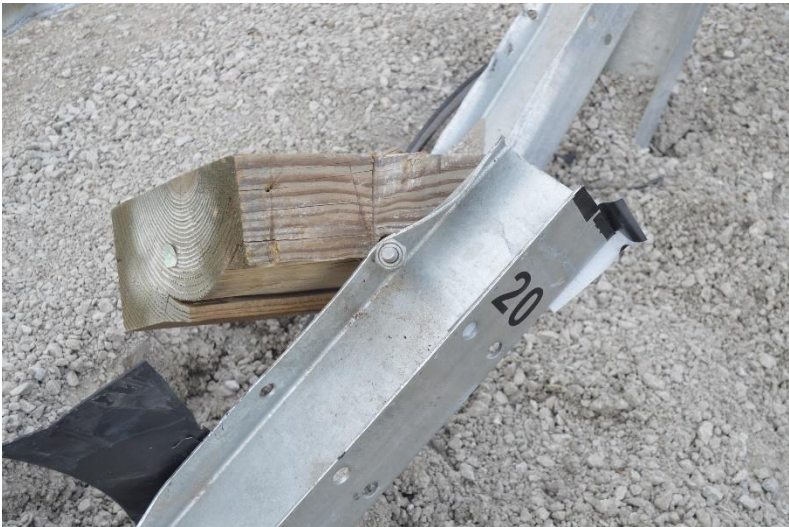
Figure 40. Bolt Hole and Bolt Damage, Post No. 20, Test No, MGS7S-1
