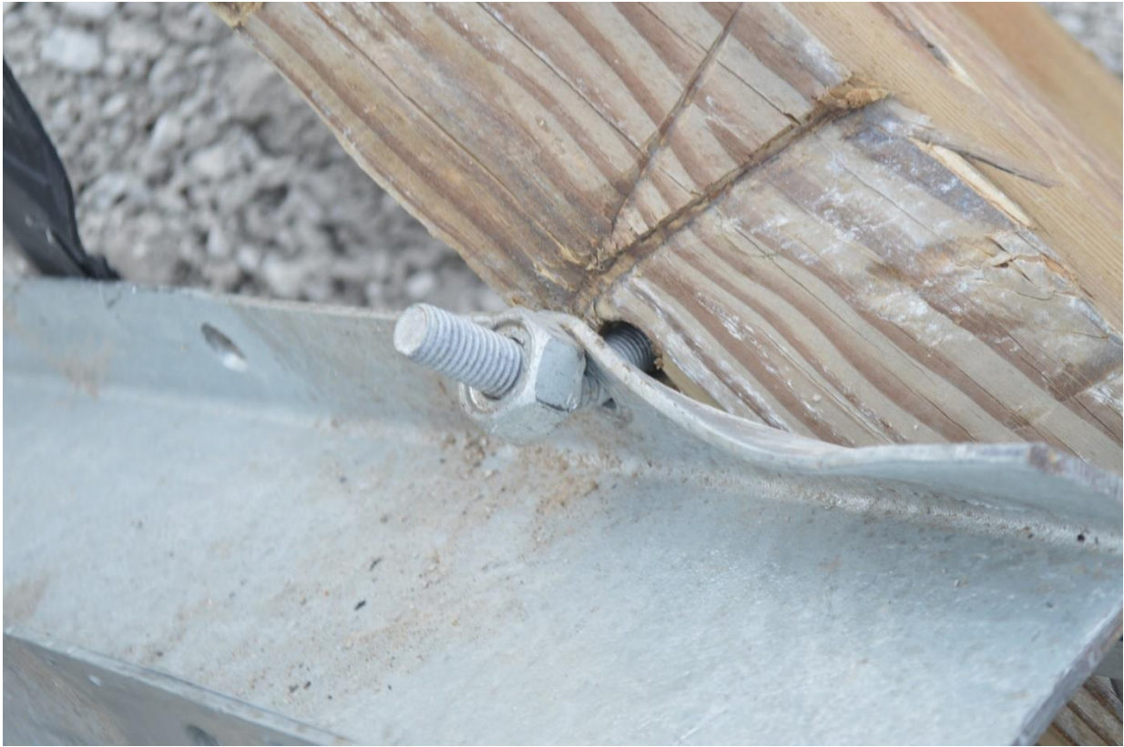
Figure 41. Bolt Hole and Bolt Damage, Test No. MGS7S-1
