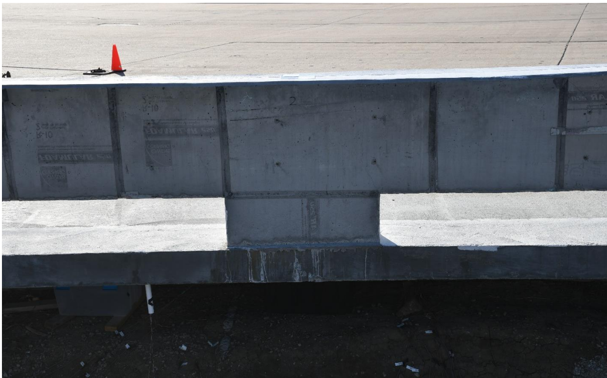
Figure 28. Typical Post Installation, Test Nos. OCBR-1, OCBR-2, and OCBR-3
