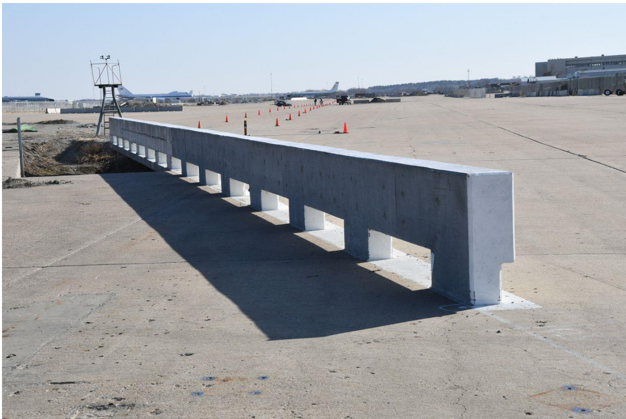
Figure 27. Test Installation Photos, Test Nos. OCBR-1, OCBR-2, and OCBR-3
