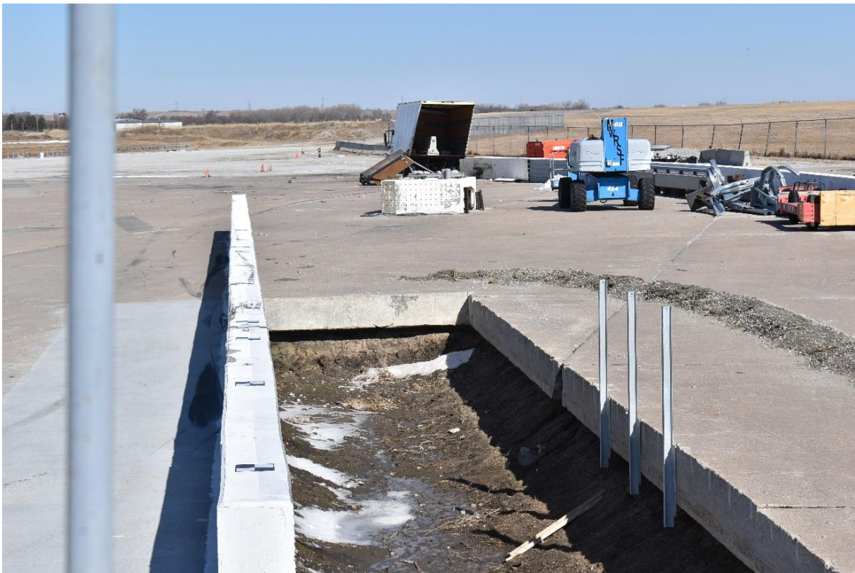
Figure 76. Vehicle Final Position and Trajectory Marks, Test No. OCBR-3
