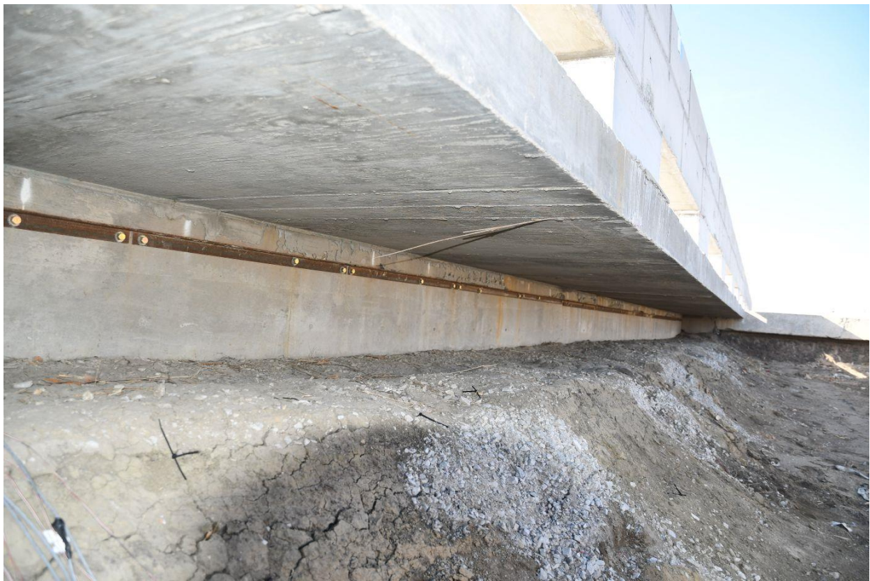
Figure 29. Bridge Deck Installation, Test Nos. OCBR-1, OCBR-2, and OCBR-3
