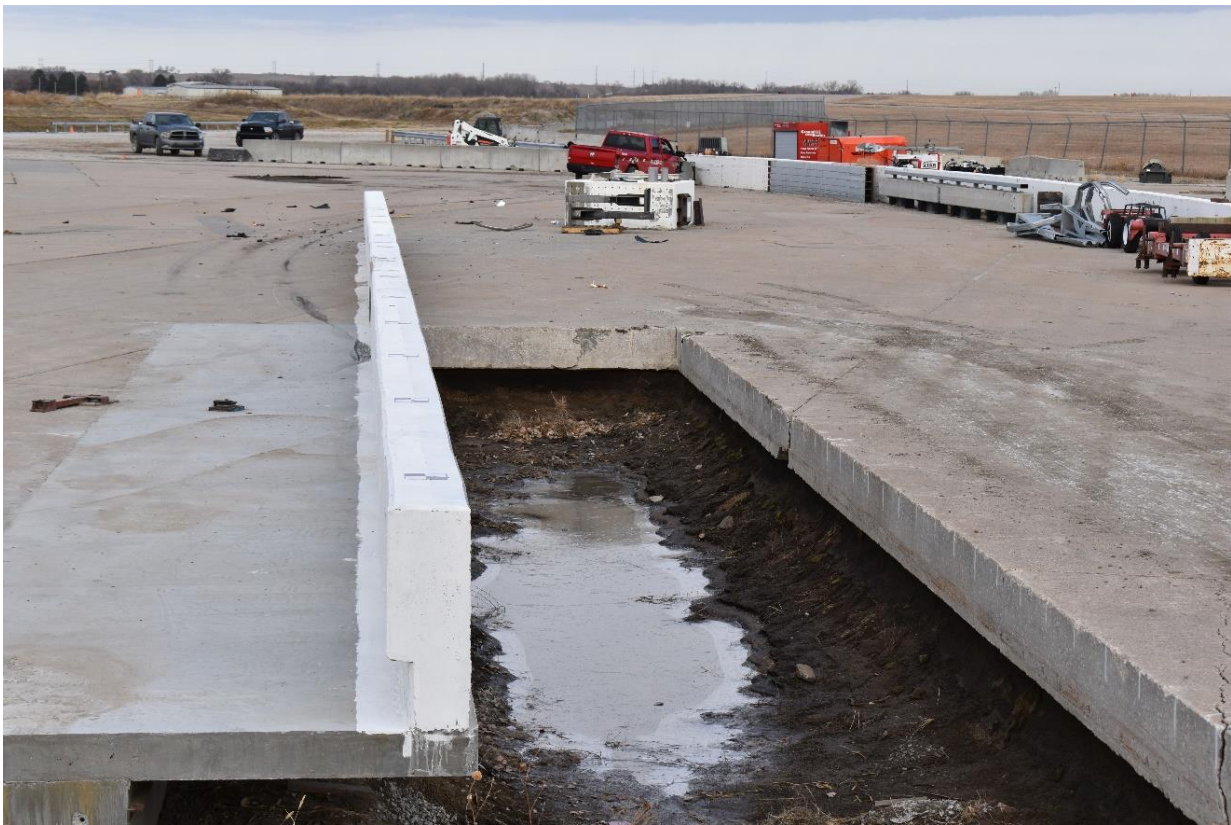
Figure 65. Vehicle Final Position and Trajectory Marks, Test No. OCBR-2
