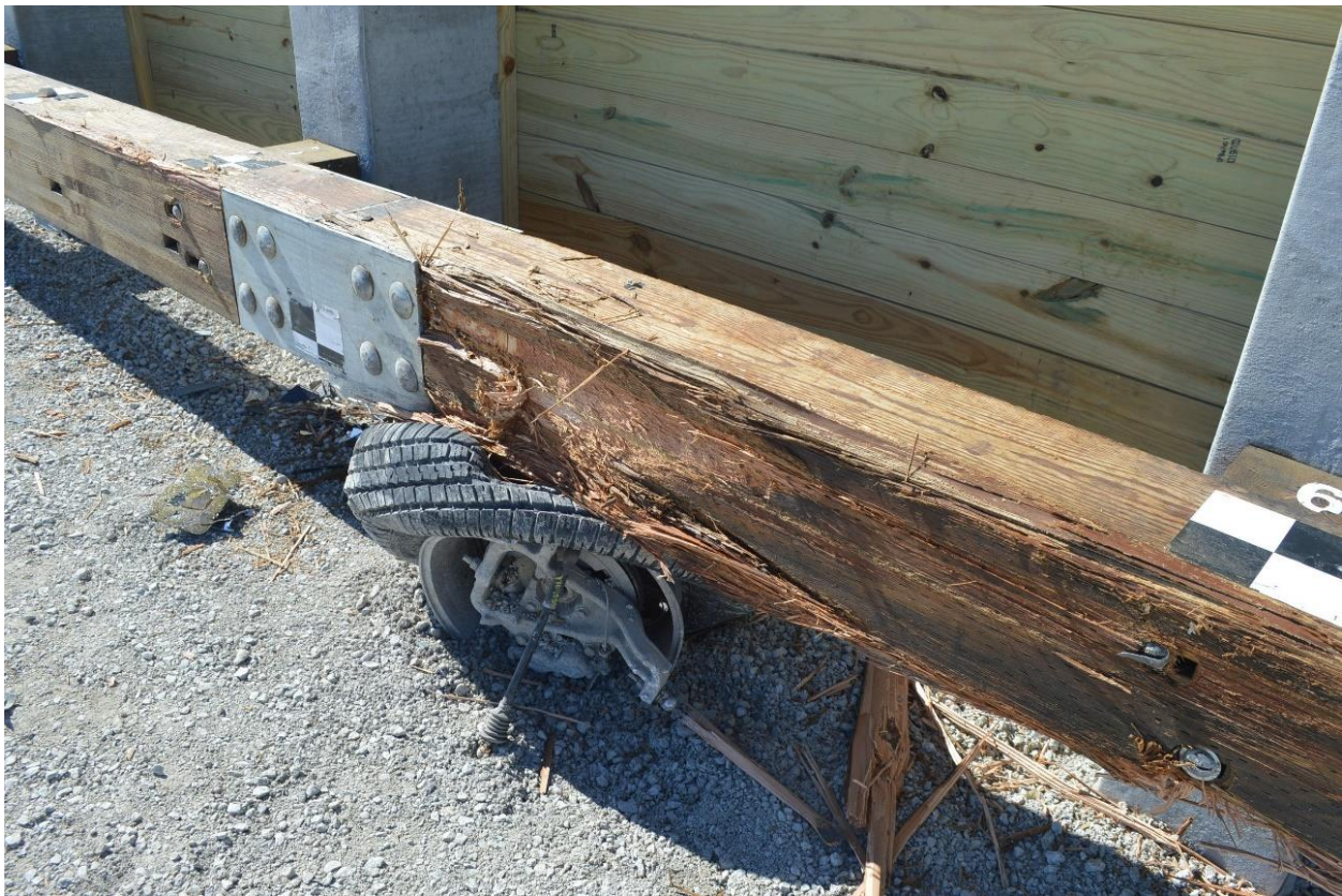
Figure 65. Lateral Extent of the 2270P Vehicle in Test No. MNNW-1 on the Minnesota Noise Wall [33]
