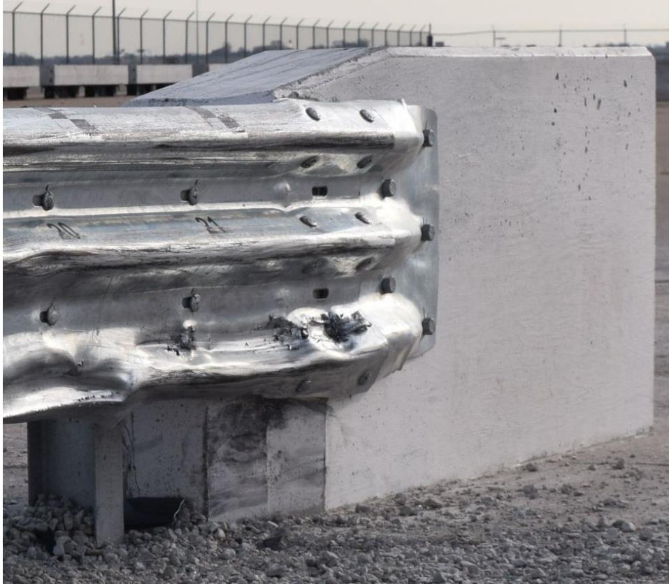
Figure 75. Lateral Extent of the 2270P Vehicle on the Standardized AGT Buttress, Test No. AGTB-1 [35]
