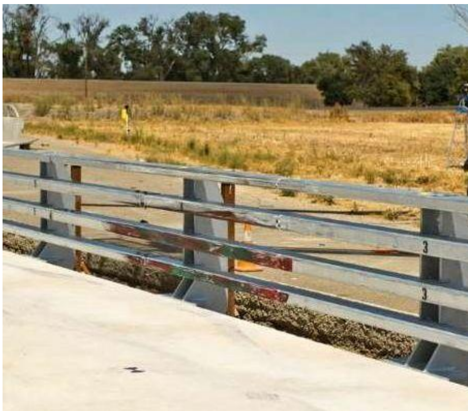
Figure 47. Lateral Extent of the 2270P Vehicle on the ST-70SM Bridge Rail [27]
