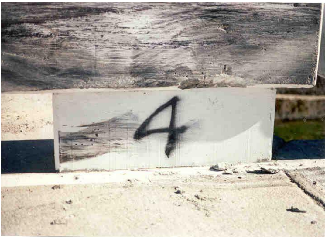
Figure 28. Lateral Extent of the 5,394-lb Pickup Truck on the Nebraska Open Concrete Rail [22]
