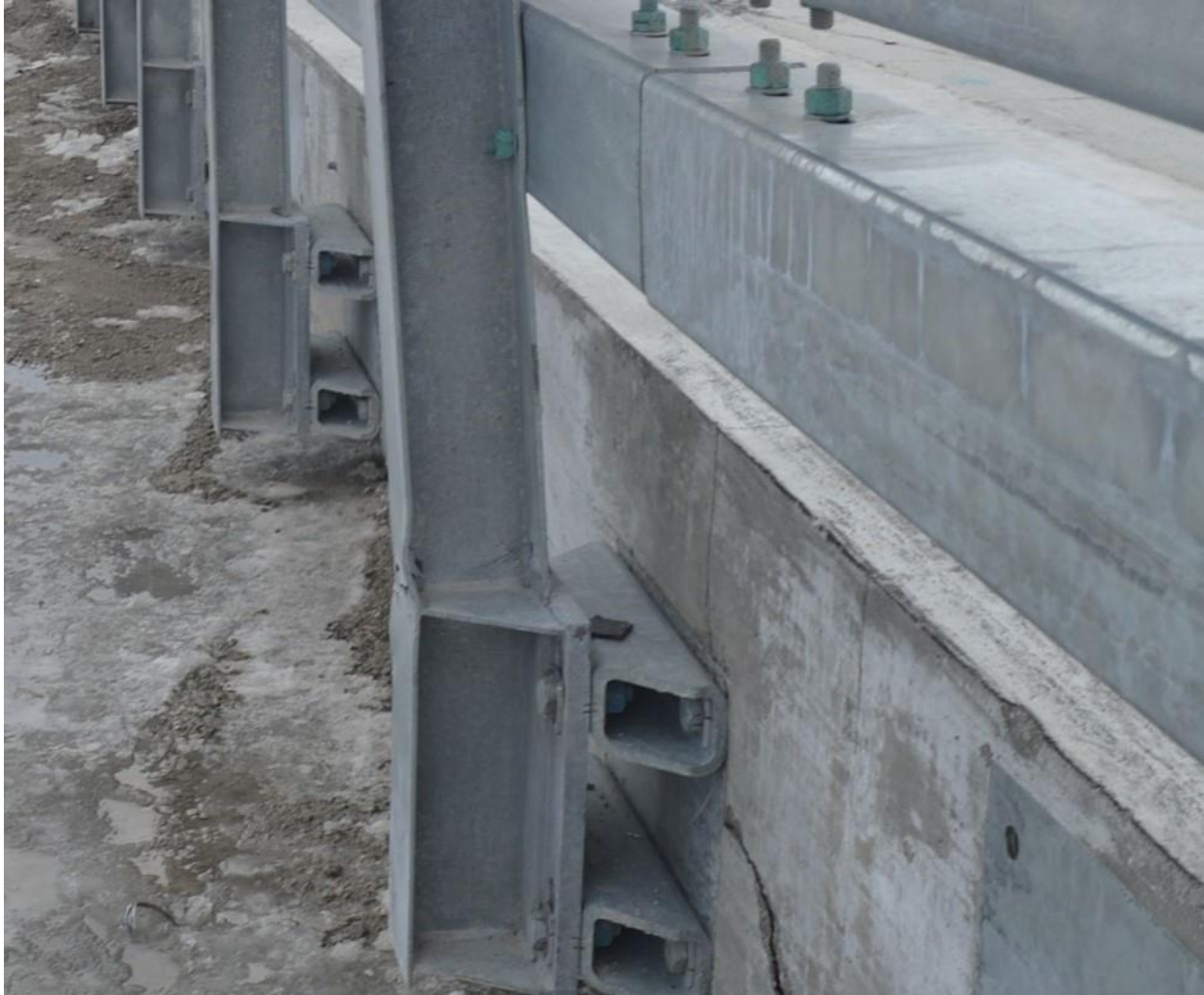
Figure 58. Lateral Extent of the 2270P Vehicle on the 36-in. Tall Illinois-Ohio Steel Bridge Rail [29-32]
