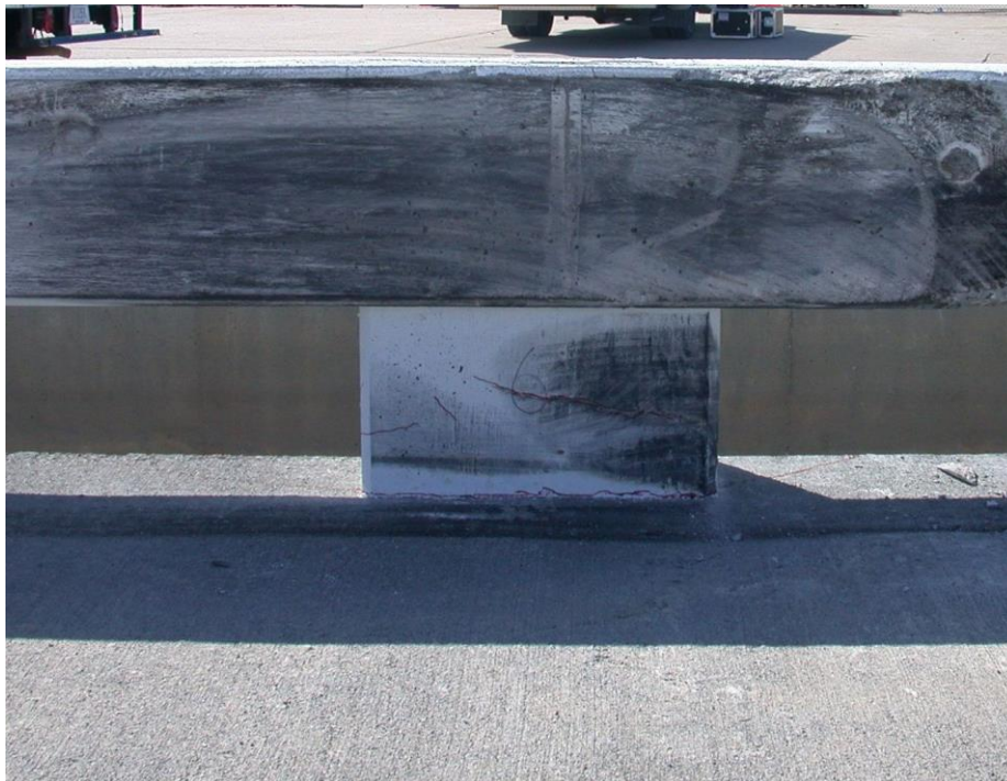
Figure 31. Lateral Extent of the 2000P Vehicle on the Nebraska Open Concrete Rail on an IT Bridge Deck [1]
