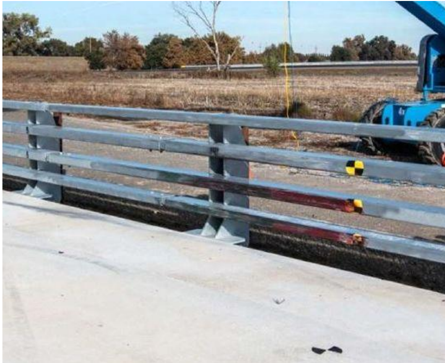
Figure 46. Lateral Extent of the 1100C Vehicle on the ST-70SM Bridge Rail [27]
