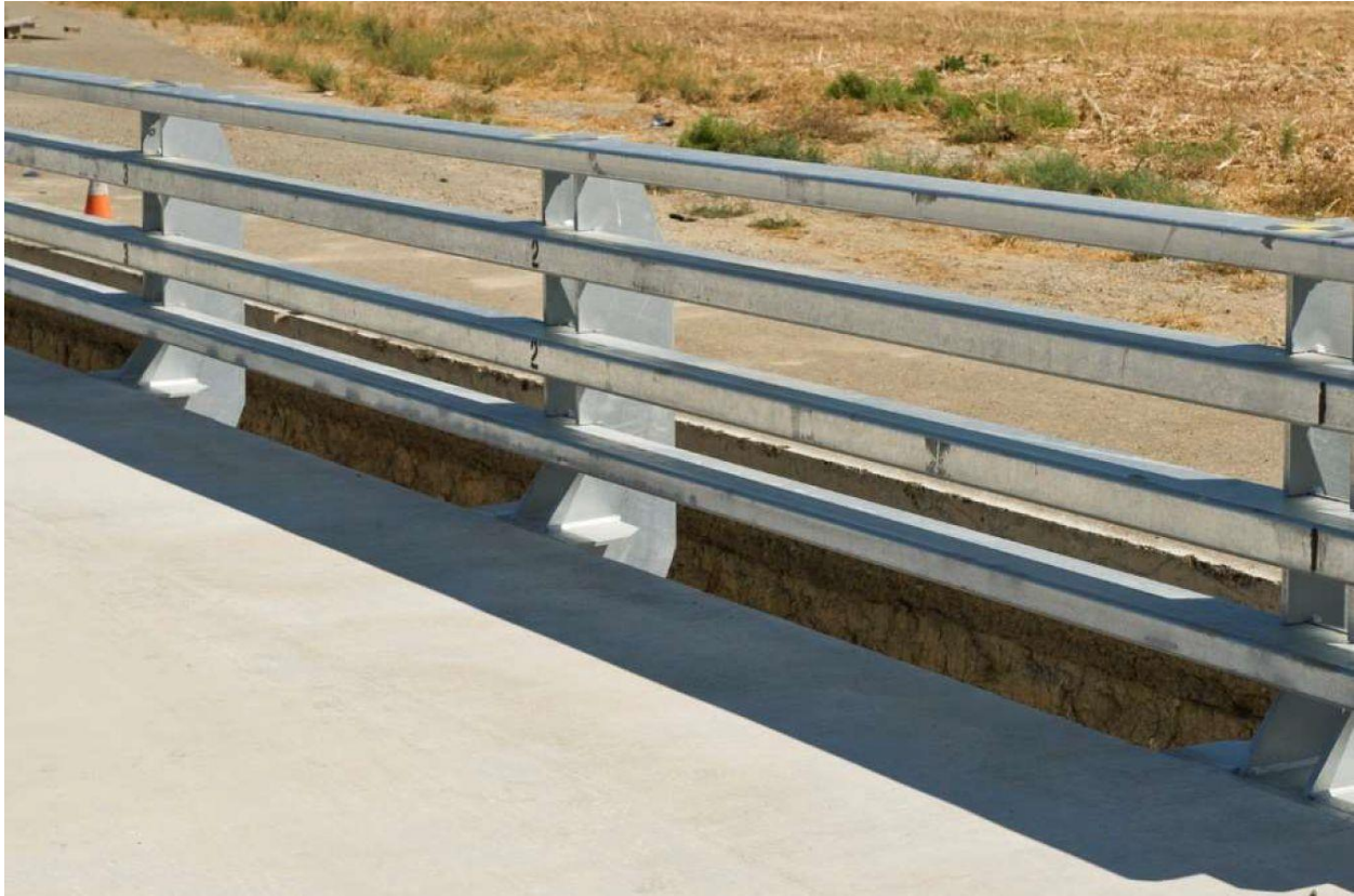
Figure 44. California ST-70SM Bridge Rail System Photograph [27]
