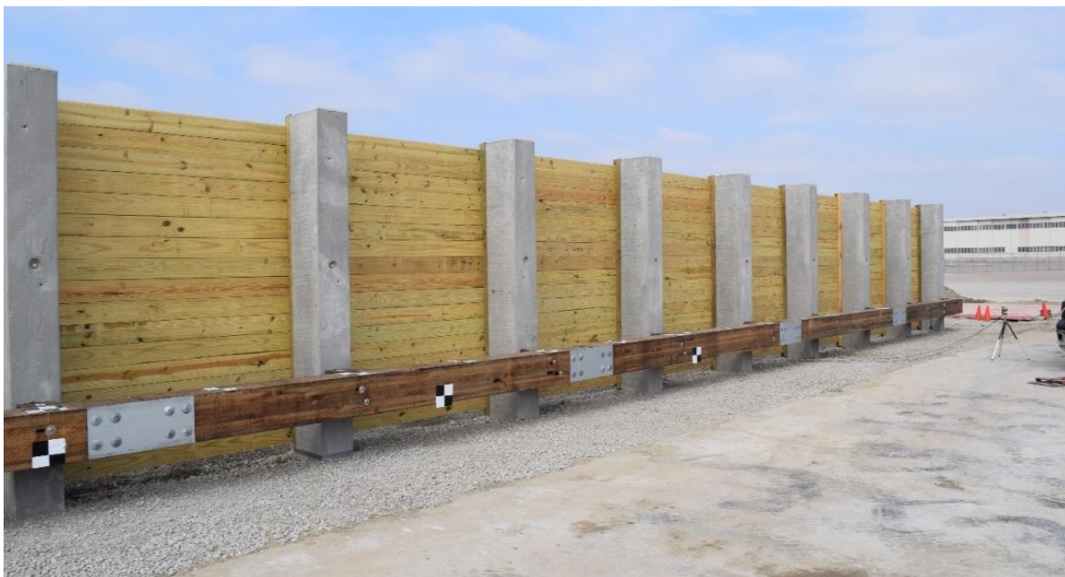
Figure 61. Minnesota Noise Wall Test Nos. MNNW-1 and MNNW-2 System Photograph [33]
