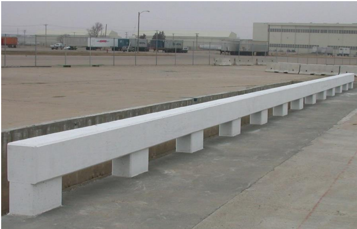
Figure 29. Nebraska Open Concrete Rail on an IT Bridge Deck System Photograph [1]
