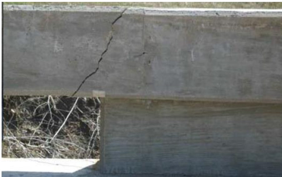
Figure 104. Open Concrete Bridge Rail Failure Mechanism [39]
