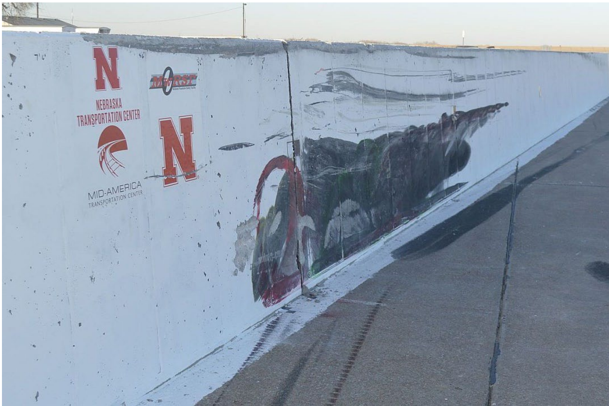
Figure 6.12 System Damage, Test No. MTL6-1
