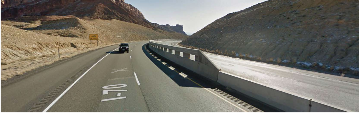
Figure 2.5 Utah DOT 84-in. Tall Roman Wall Installation [3]
