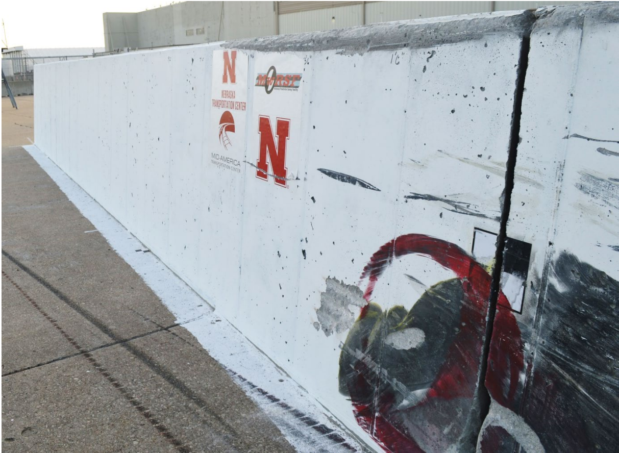
Figure 6.14 System Damage Near Expansion Joint, Test No. MTL6-1
