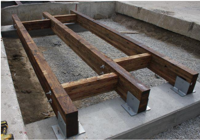
(c) Construction of Glulam Girders and Diaphragms
