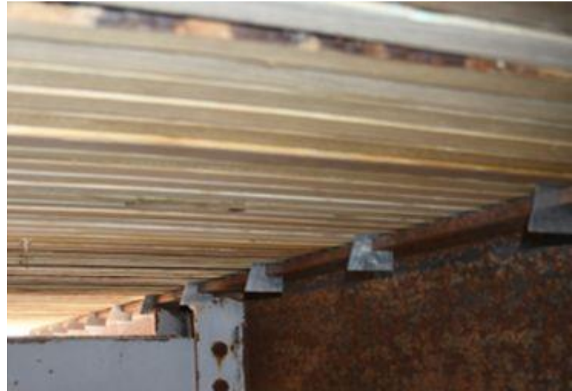
(b) Anchor Brackets on Underside of Nail-Laminated Deck
