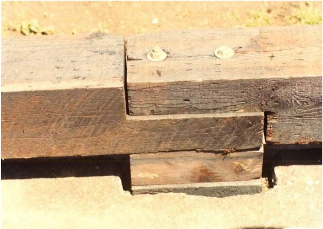
(b) Lap Splice Connection
