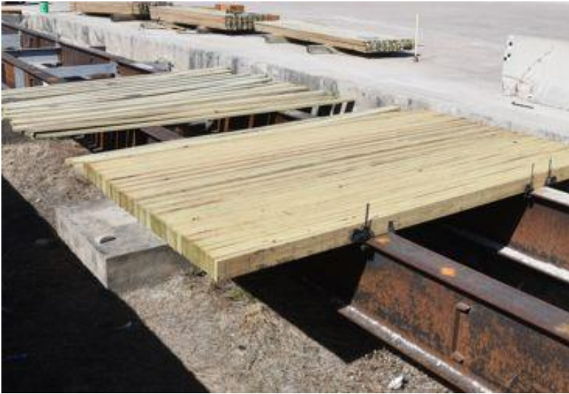
(a) Construction of Nail-Laminated Deck
