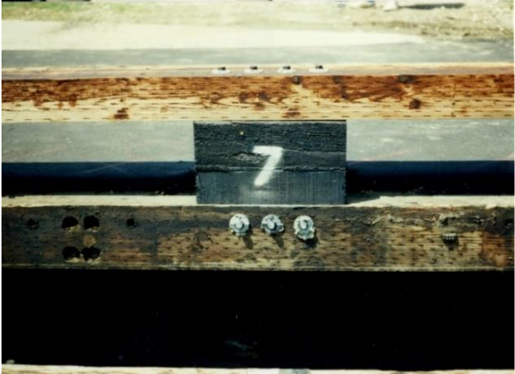
(a) Scupper Block and Glulam Rail Connection
