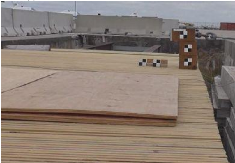
(c) Side View of Nail-Laminated Deck
