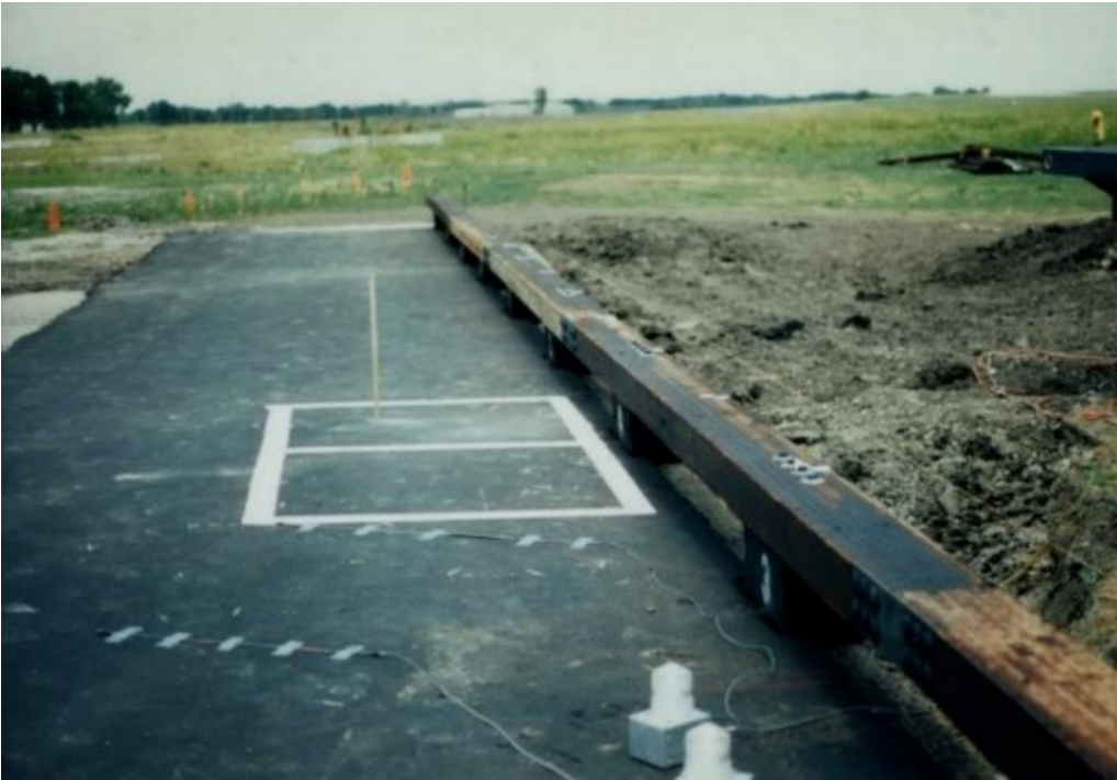
(b) Upstream End View
