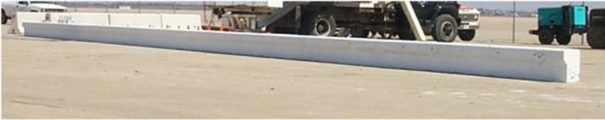
Figure 2. Constructed TL-2 Low-Profile, Concrete Bridge Rail System for Full-Scale Crash Testing [2]
