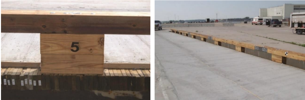
Figure 11. Low-Height, Curb-Type, Glulam Bridge Railing [5-6]
