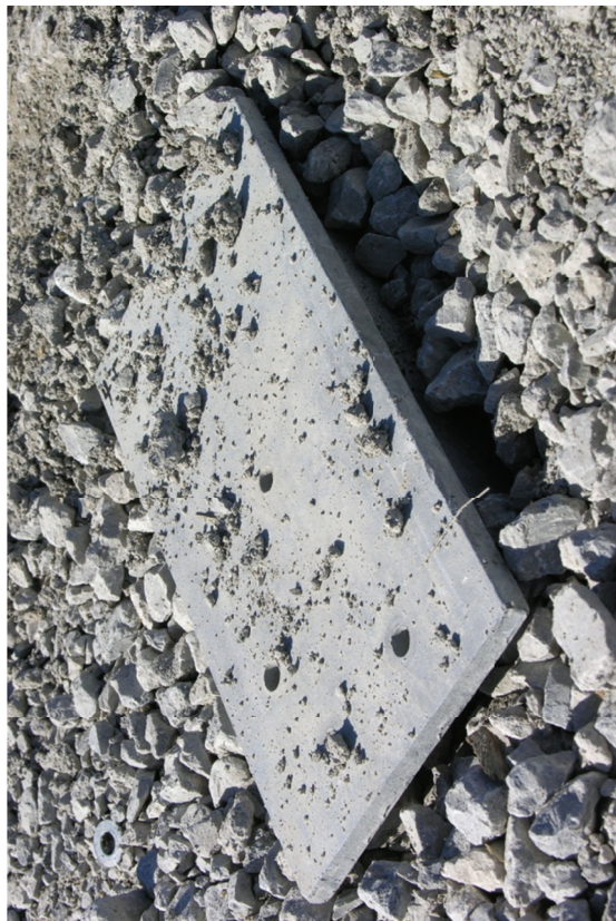
Figure 53. Post Damage, Test No. USPN-4
