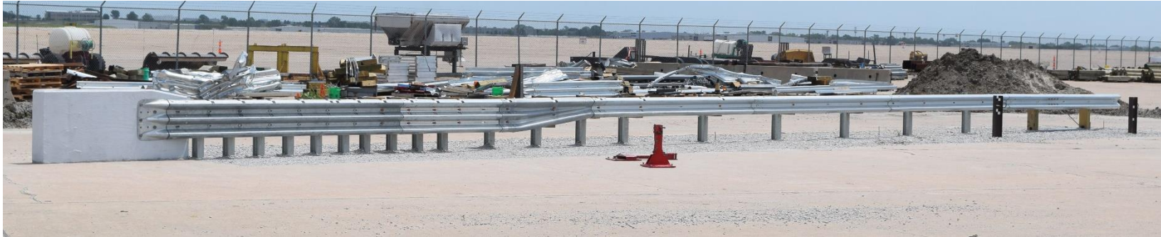
Figure 1. AGTB-2 Guardrail Installation
