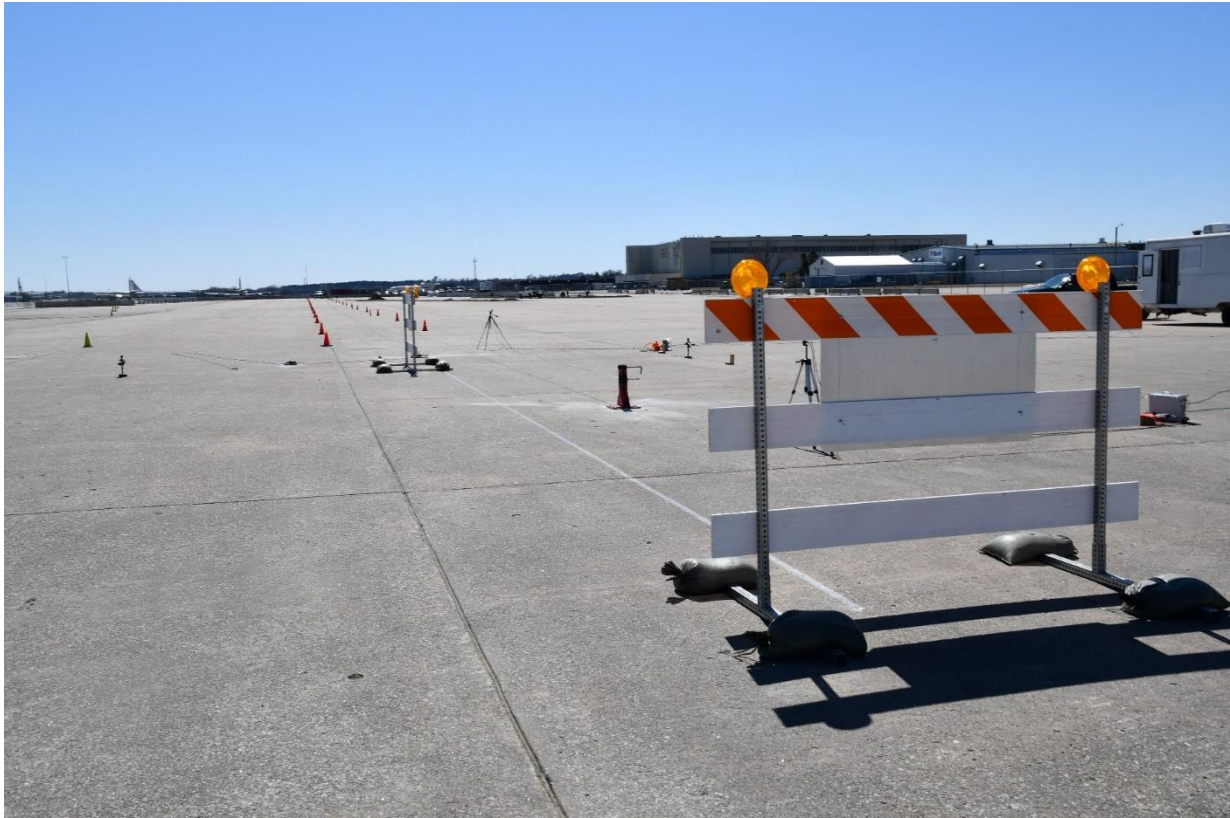
Figure 9. Test Installation, Test No. WZNP-2
