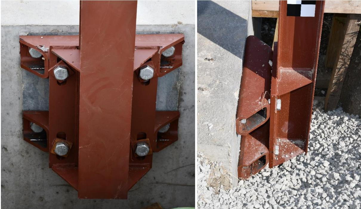
Figure 9. Photos of Assembled Post-to-Deck Connection [12]
