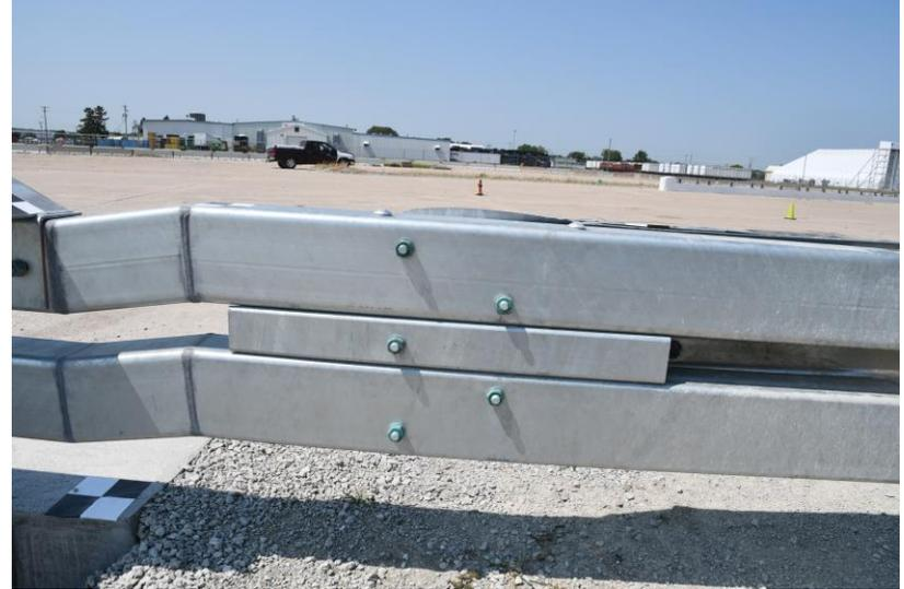
Figure 19. Photographs of the AGT to Steel Railing, Type IL-OH
