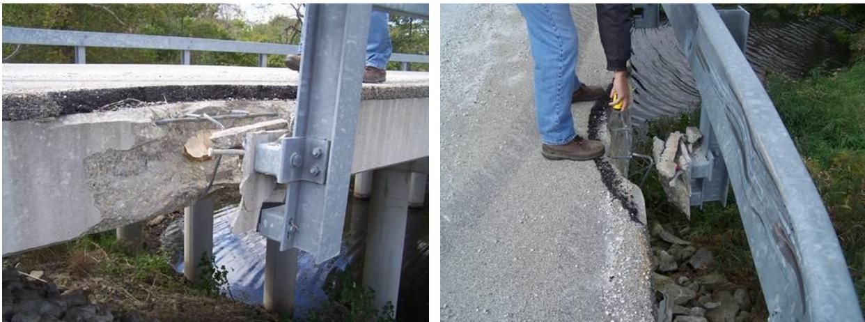
Figure 5. Post-to-Deck Anchorage Failure of Previous Connection Design
