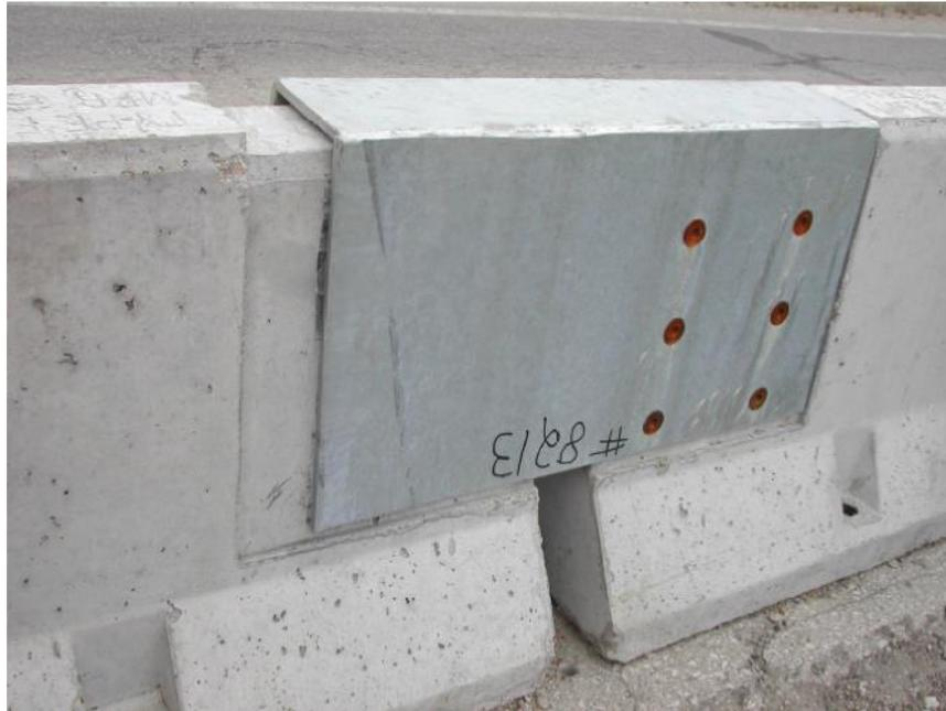
Figure 15. Example of Steel Cover Plate at Expansion/Contraction Joints
