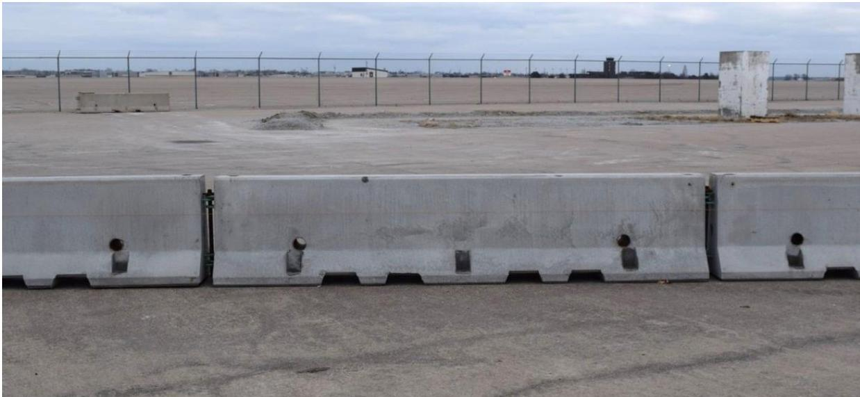
Figure 1. Free-Standing, F-Shape, Portable Concrete Barrier
