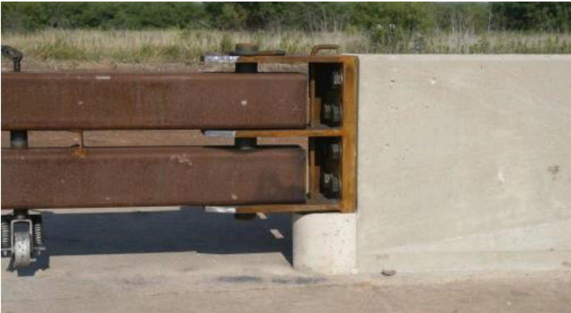
Figure 5. Original MASH TL-3 Emergency Opening System [13]
