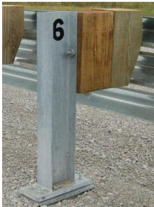
Figure 11. UBSP in Thrie-Beam Bullnose System [1]
