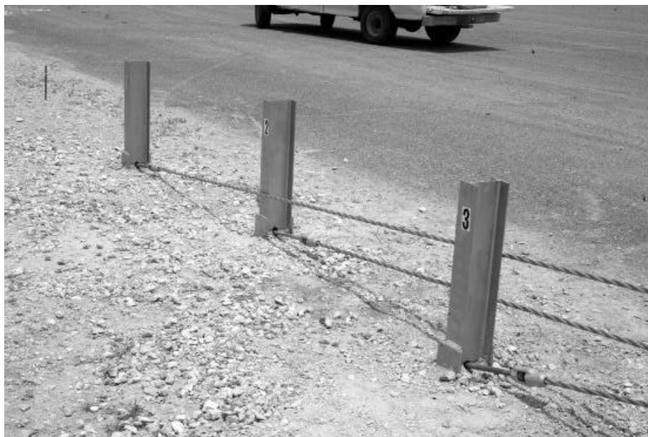
Figure 21. TTI End Terminal [39]
