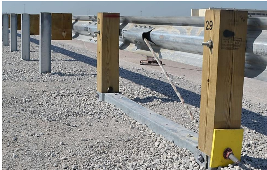
Figure 2. MGS Trailing-End, Guardrail Anchorage System [4]
