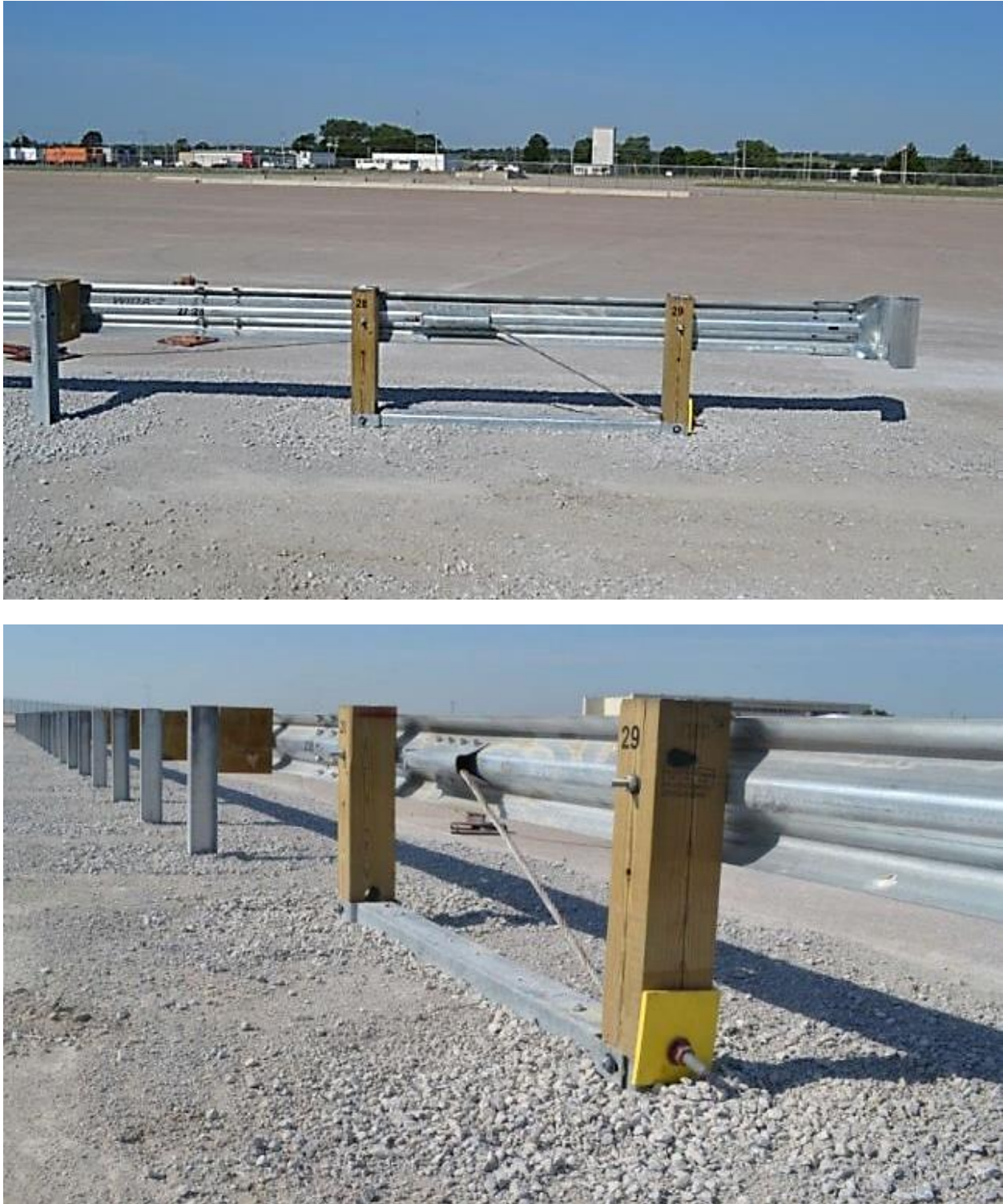
Figure 9. MGS Trailing-End Anchorage System [4]
