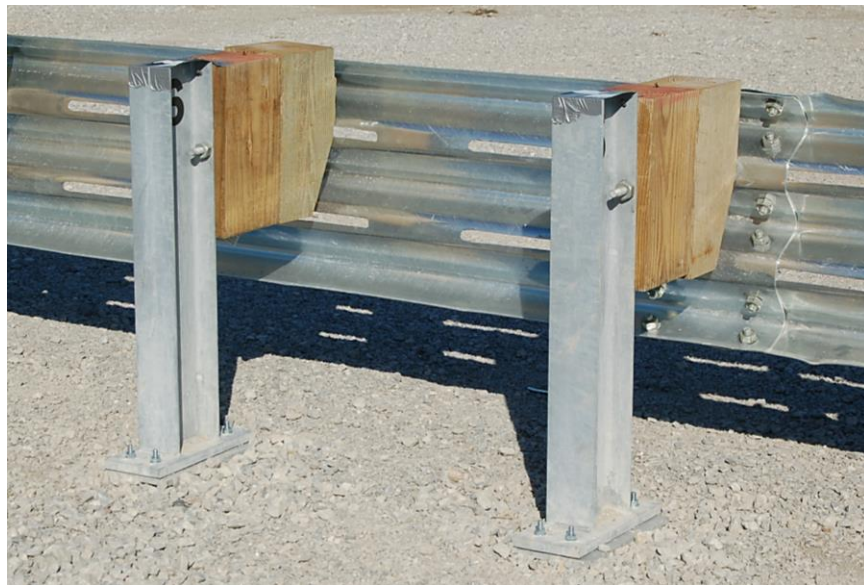
Figure 1. UBSP Utilized in Thrie Beam Bullnose System [2]
