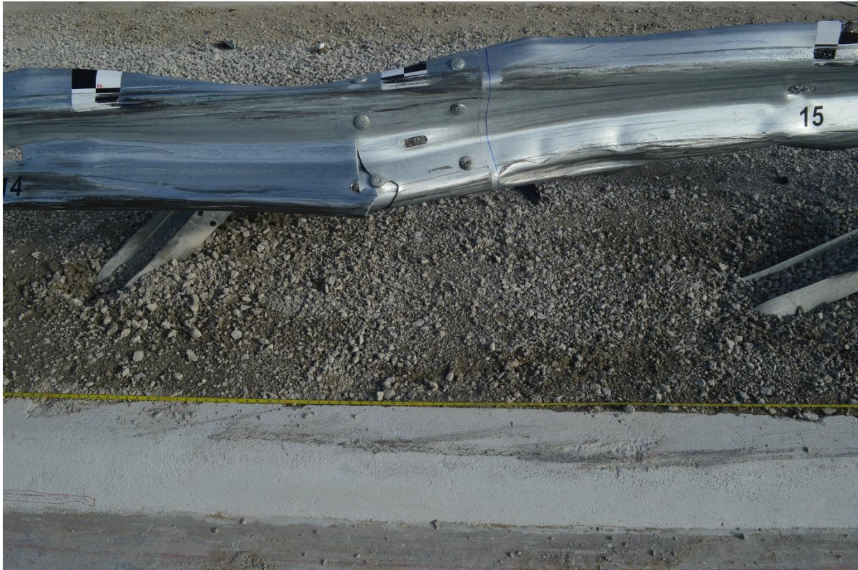
Figure 57. Curb Damage, Test No. MGSC-7
