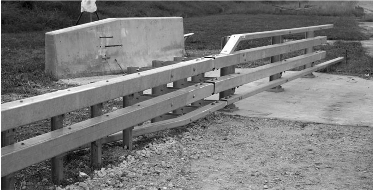
Figure 44. Box Beam Transition to Four-Tube Steel Bridge Rail [24]
