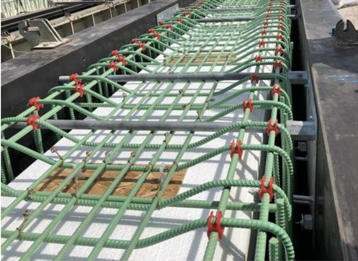
Figure 61. Reinforcement and Post Anchorage Placement Prior to Casting
