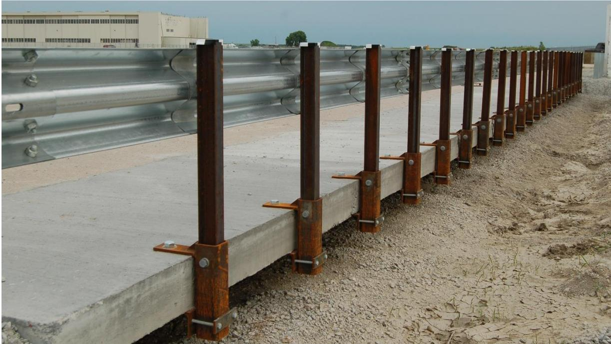
Figure 21. Weak-Post Midwest Guardrail System [28]
