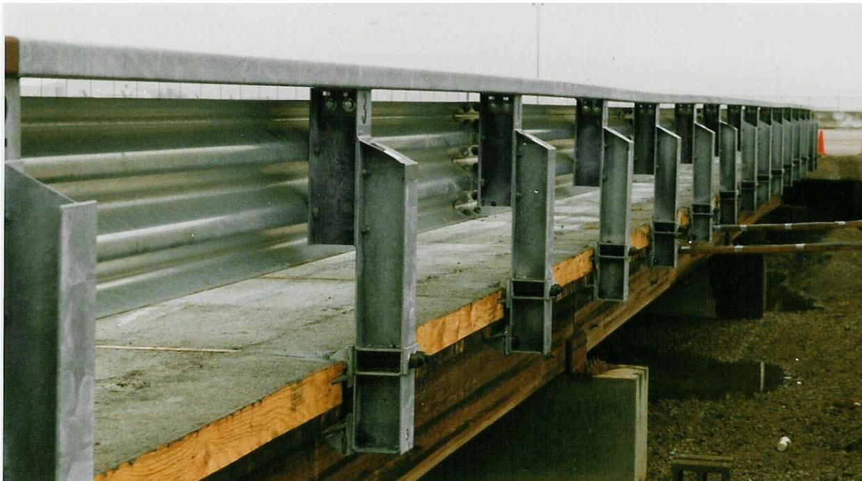
Figure 20. TL-4 Thrie-Beam Bridge Rail for Timber Decks [27]
