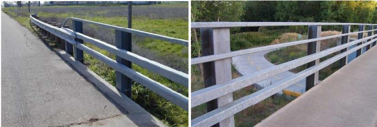
Figure 9. California Type 116 and 117 Bridge Rails [18]
