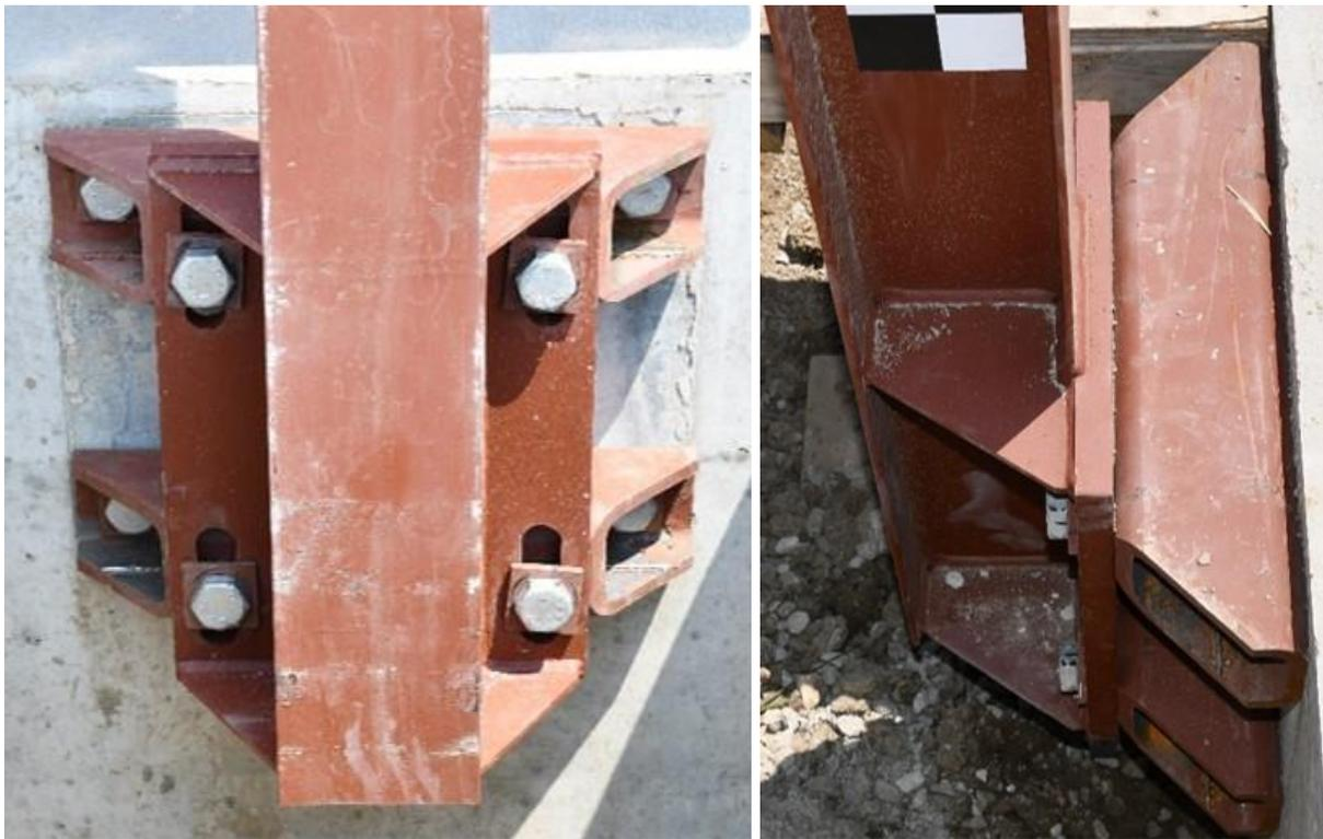
Figure 125. Post-to-Deck Connection Final Design
