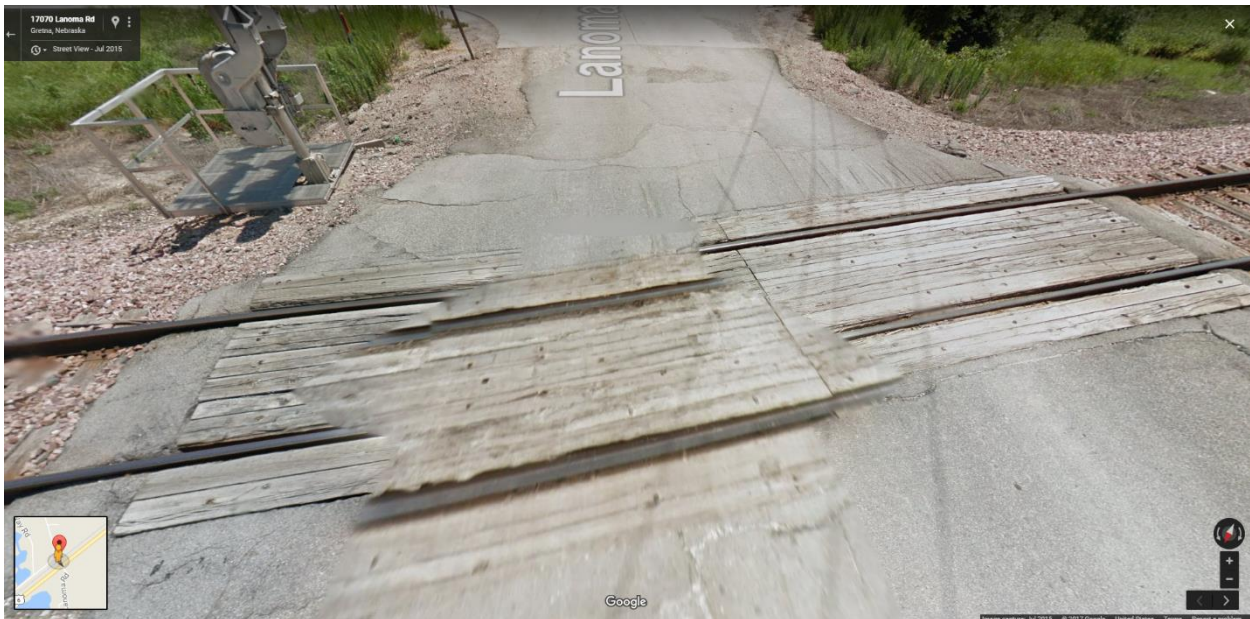
Figure 82. Google Street View of Scrape Marks on Crossing 073158N [49]
