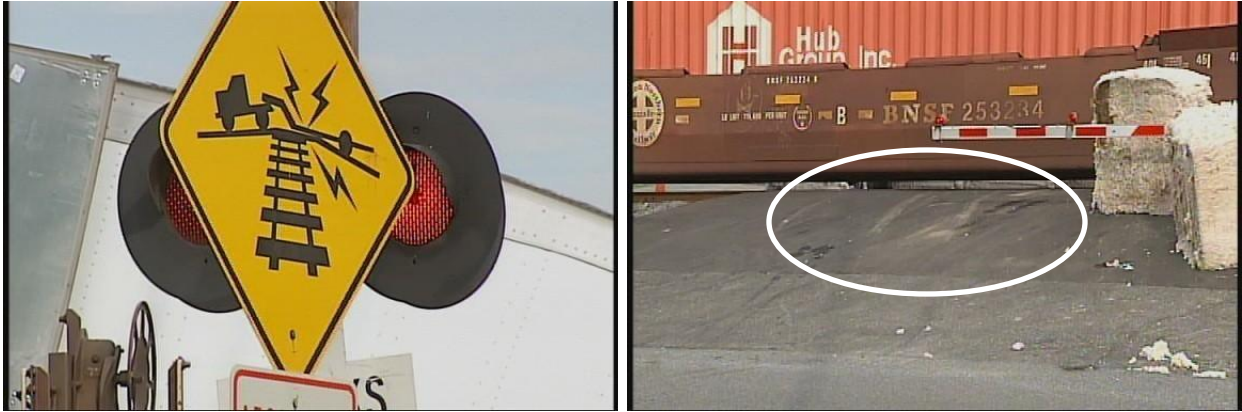
Figure 38. Rail Grade Crossing Warning and Scrape Marks at Grade Crossing [35]
