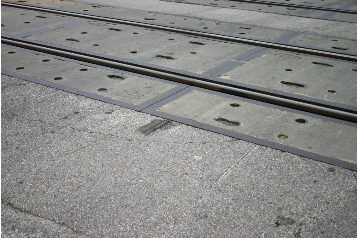
Figure 100. West Approach of Crossing 816134F with Scrape Marks on the Asphalt, Close Up
