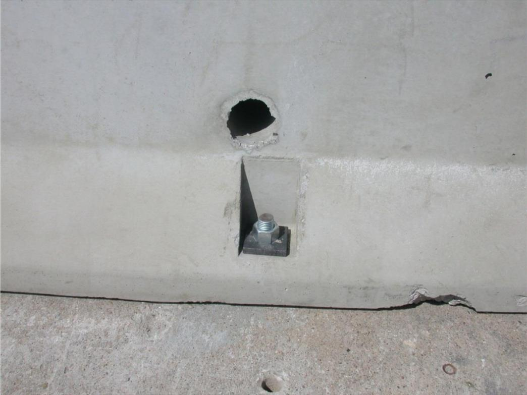
Figure 1. Bolt-Through Tie-Down for F-Shape PCB
