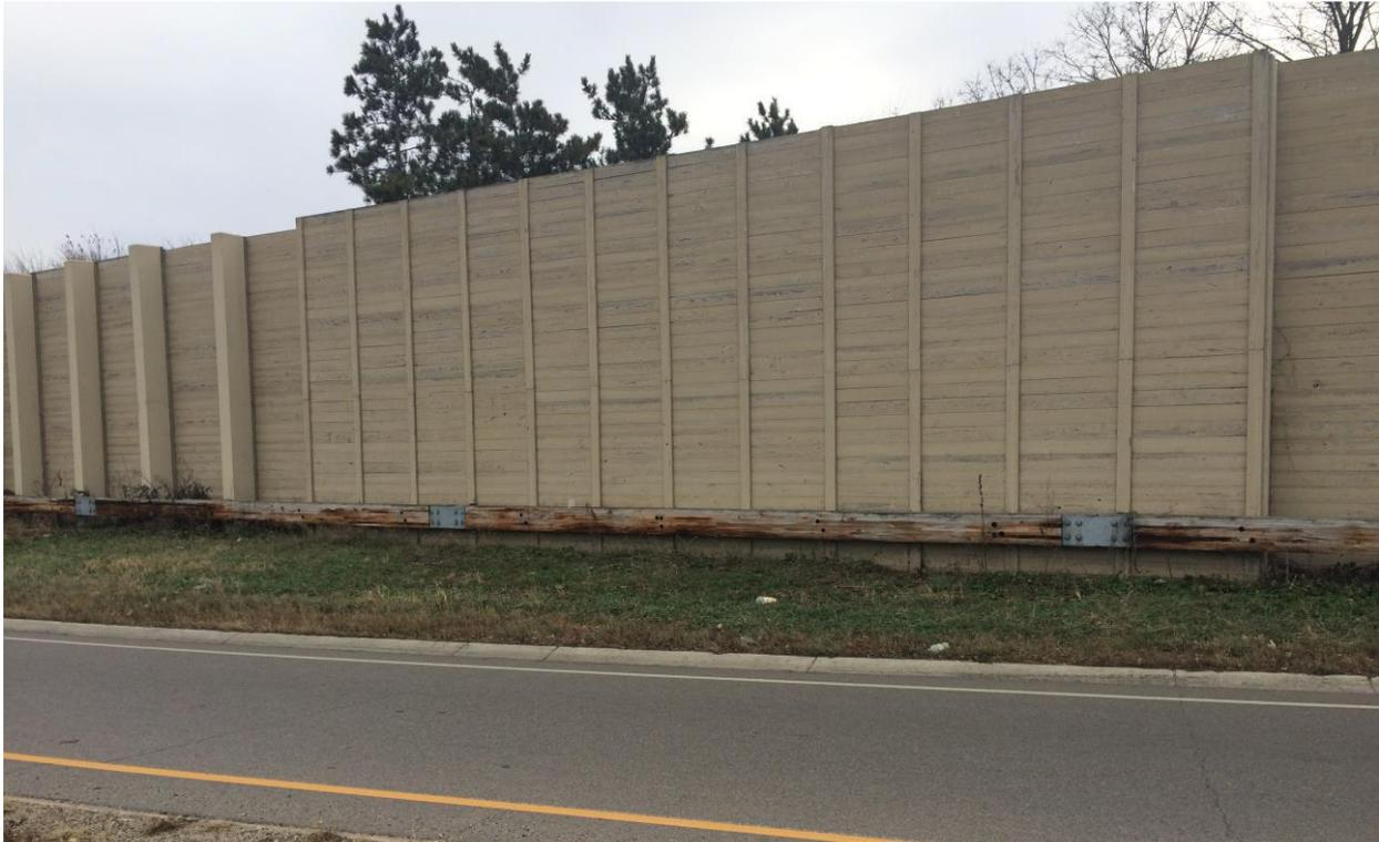
Figure 1. MnDOT Noise Wall and Rubrail Installation
