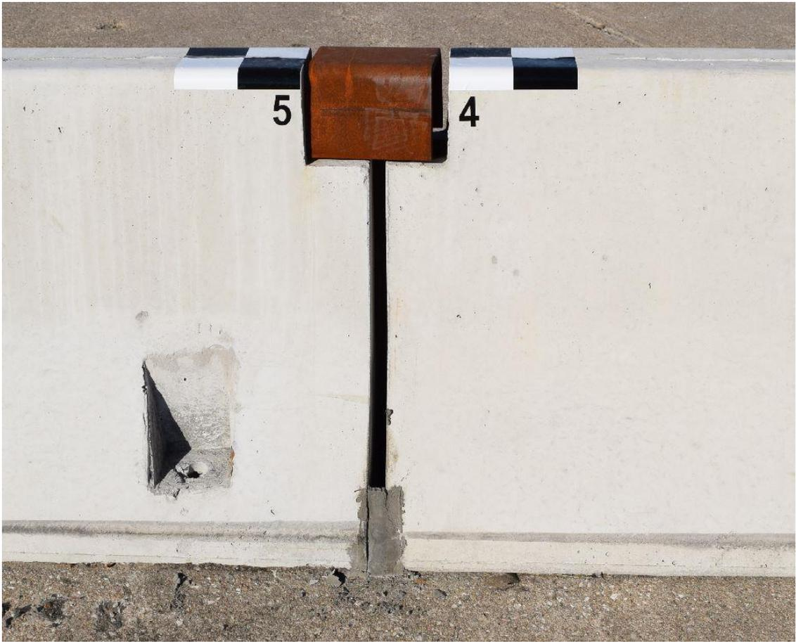
Figure 16. PCB Connection Key, Connection Socket, and Grout at Toes Between Barriers, Test No. NJPCB-4
