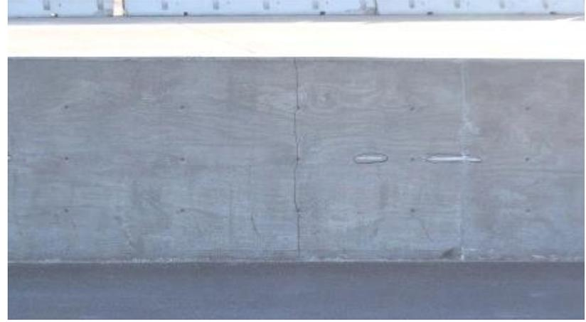
Barrier No. 5 Thermal Hairline Crack
