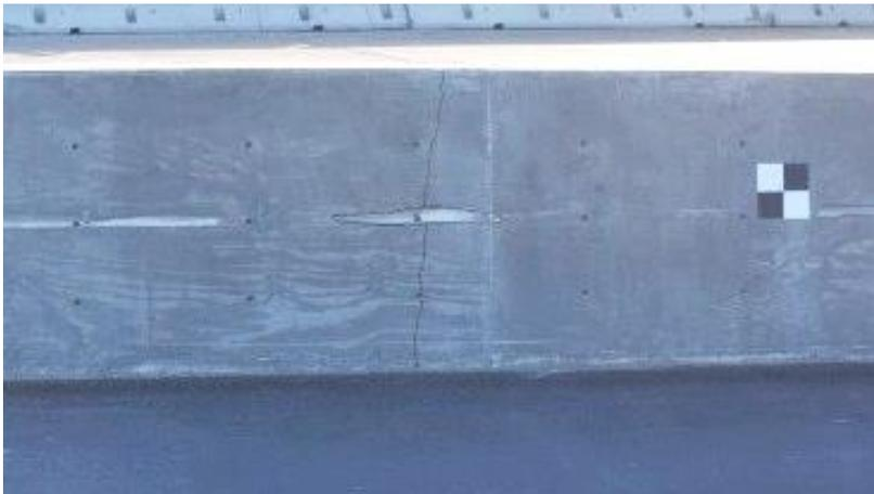
Barrier No. 2 Thermal Hairline Crack
