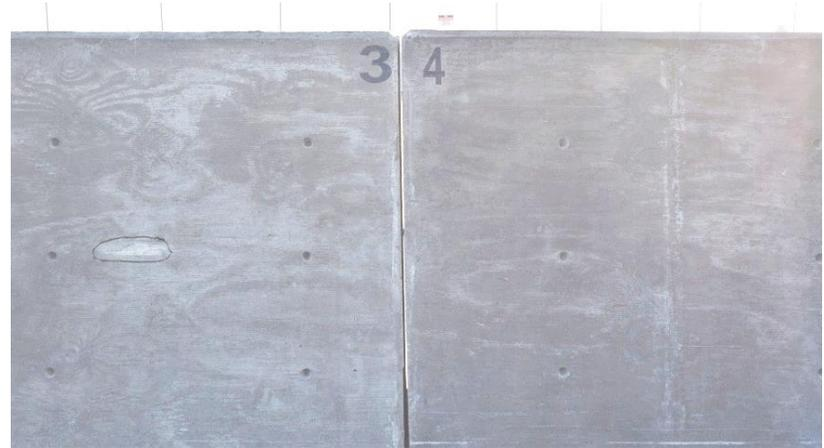
Spalling of Barrier Gap
