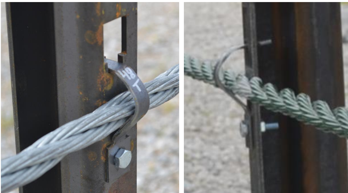
Figure 1. Bolted, Tabbed Bracket on MWP
