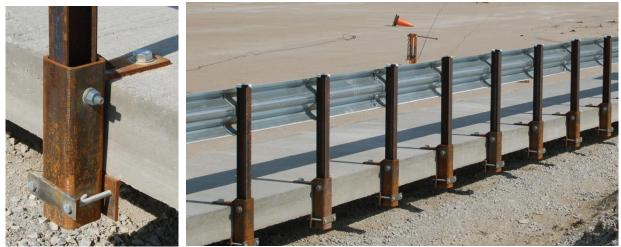
Figure 2. MGS Bridge Rail Installation
