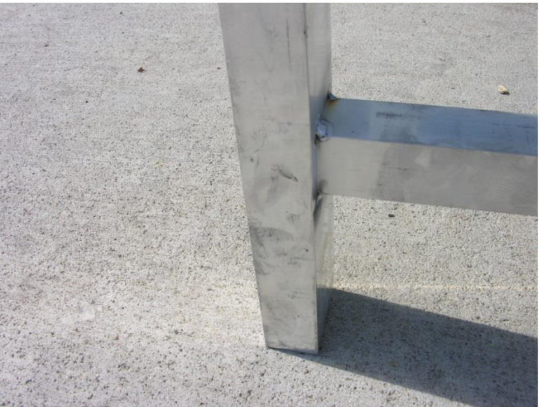
Figure 48. Welded Aluminum Rail, Design Concept AW2
