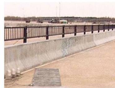
Figure 4. Concrete Traffic/Pedestrian Rail
