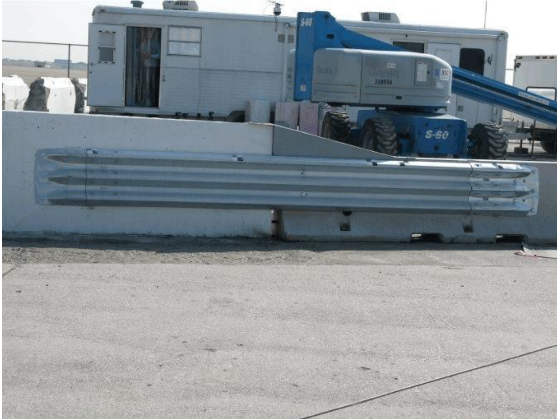
Figure 11. Transition from PCB to Permanent Concrete Barrier [2]
