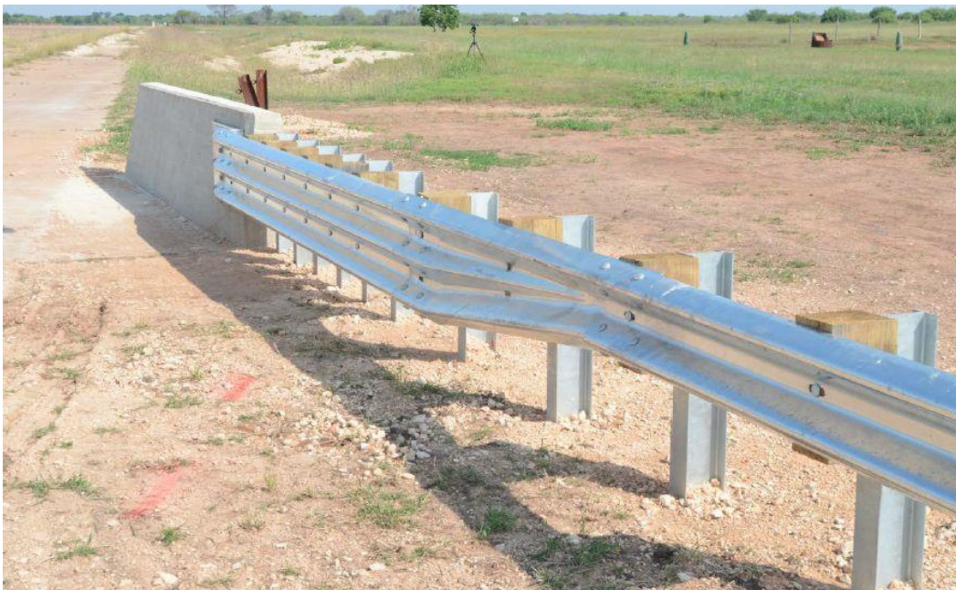
Figure 20. Thrie Beam Transition without Curb [23]
