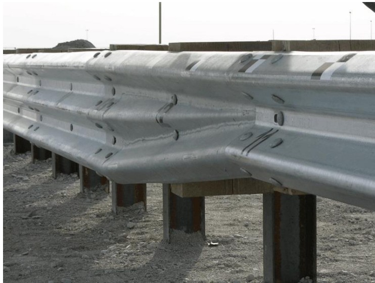
Figure 19. MGS Stiffness Transition with Asymmetrical Element [21]
