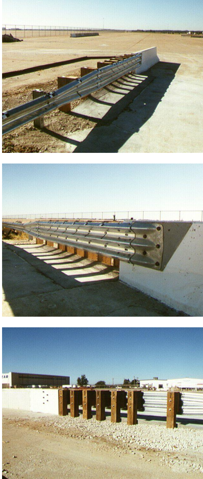
Figure 2. Generic W-Beam-to-Thrie Beam-to-Concrete Bridge Rail Transition
