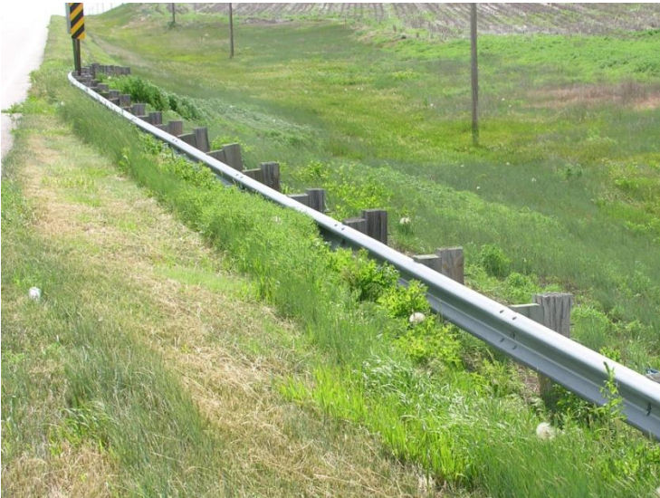
Figure 15. Examples of Low Heights for Existing W-beam Guardrail Systems
