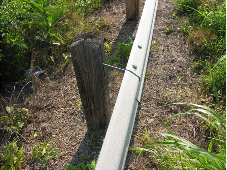
Figure 20. Examples Missing Blockouts in Existing Systems
