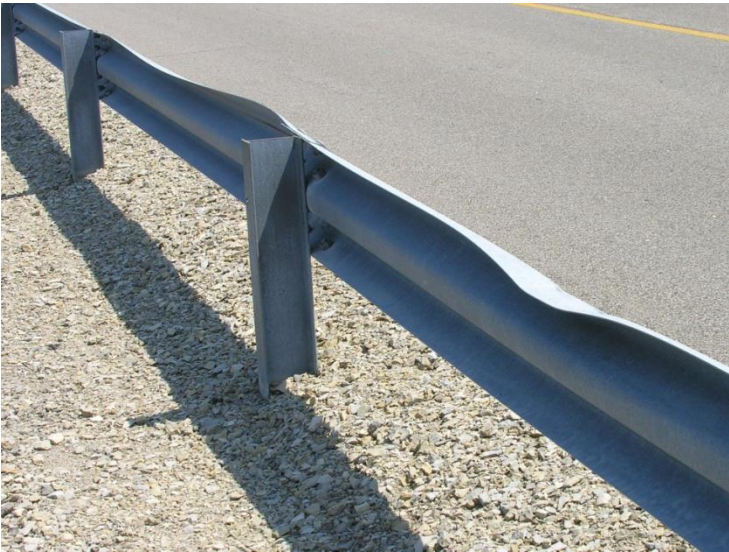
Figure 17. Examples of Rail Damage in Existing W-Beam Guardrail Systems
