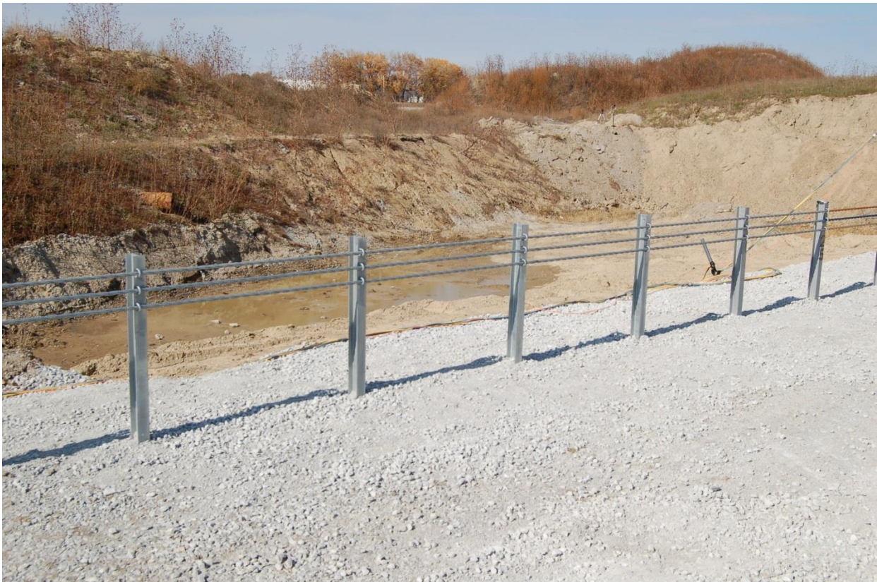
Figure 3. Generic Three-Cable Low-Tension Barrier
