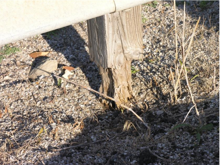
Figure 18. Examples of Missing and Inadequate Posts
