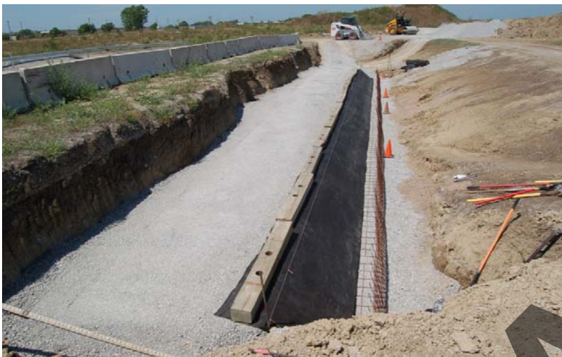
a. Filter Fabric Held by Posts
