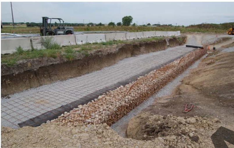
a. Second Layer Wire Mat Installed
