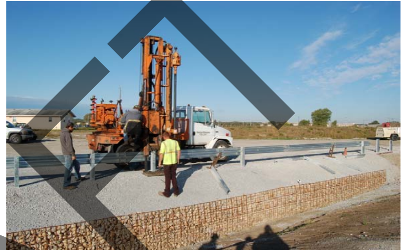
c. Non-Blocked MGS Installation, Driving Post No. 4
