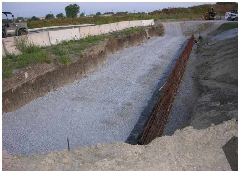
a. MSE Wall, Second Layer, Uncompacted
