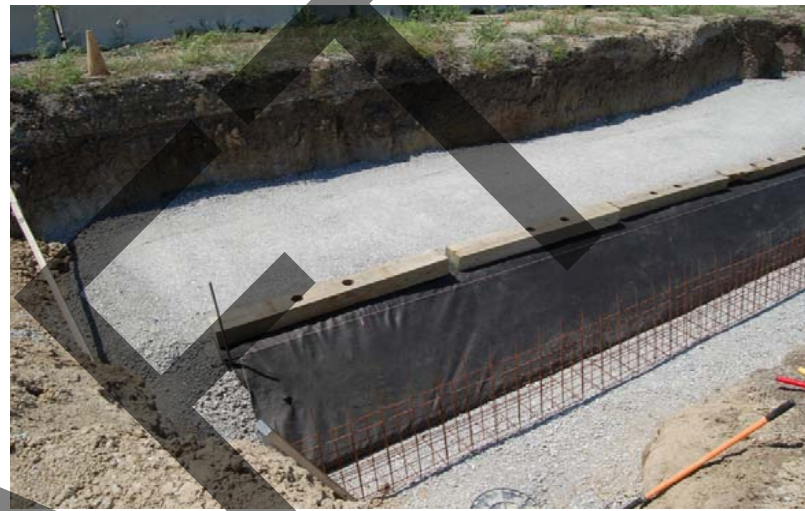
c. Filter Fabric Positioned
