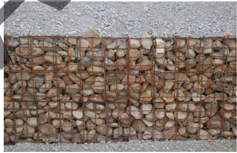
d. MSE Wall, Course Aggregate Close-up
