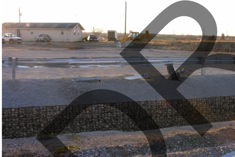
b. Impacted Rail Rear View
