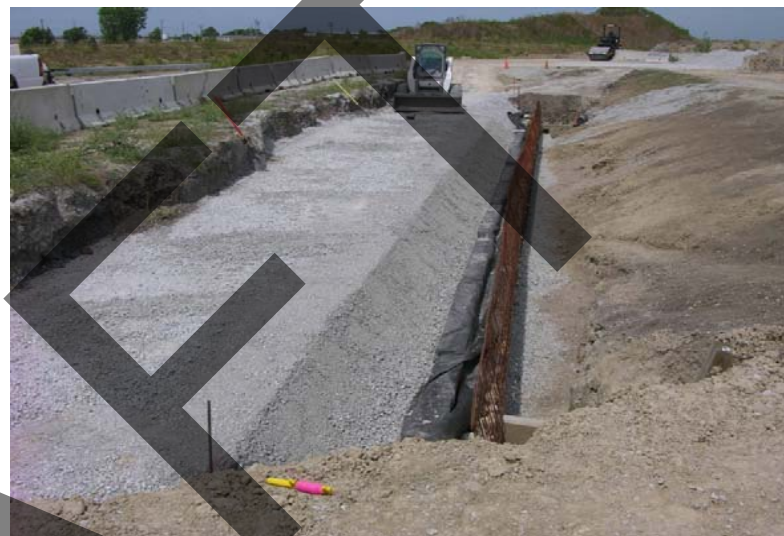
c. MSE Wall, Second Layer, Leveling
