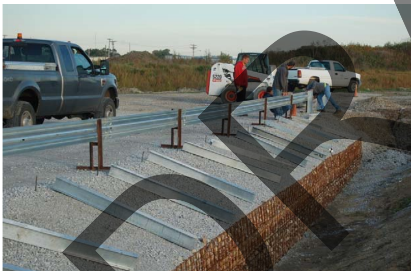
b. Non-Blocked MGS Installation, Leveling Rail
