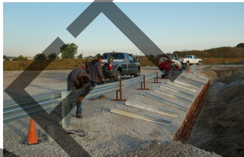
c. Non-Blocked MGS System, Initial Rail Attachment
