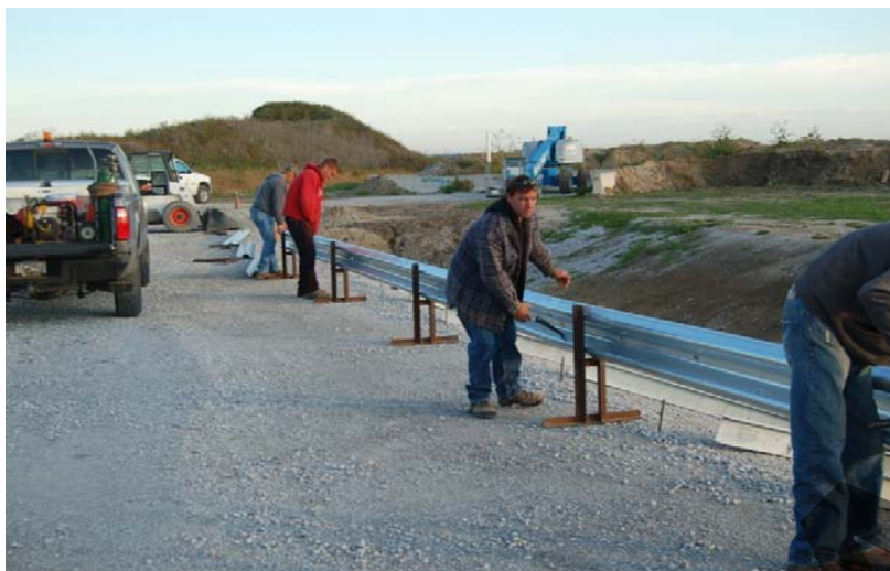
a. Non-Blocked MGS System Installation
