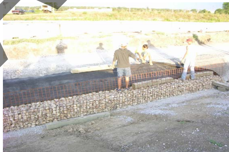
d. Second Layer Fiber Filter Positioning
