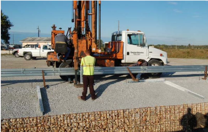
a. Non-Blocked MGS Installation, Driving Post No. 2
