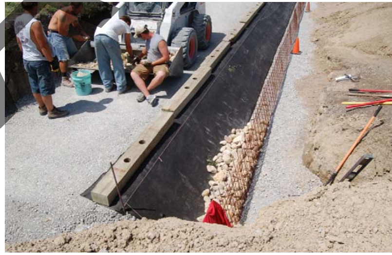
d. Wall Face Aggregate Filled by Hand
