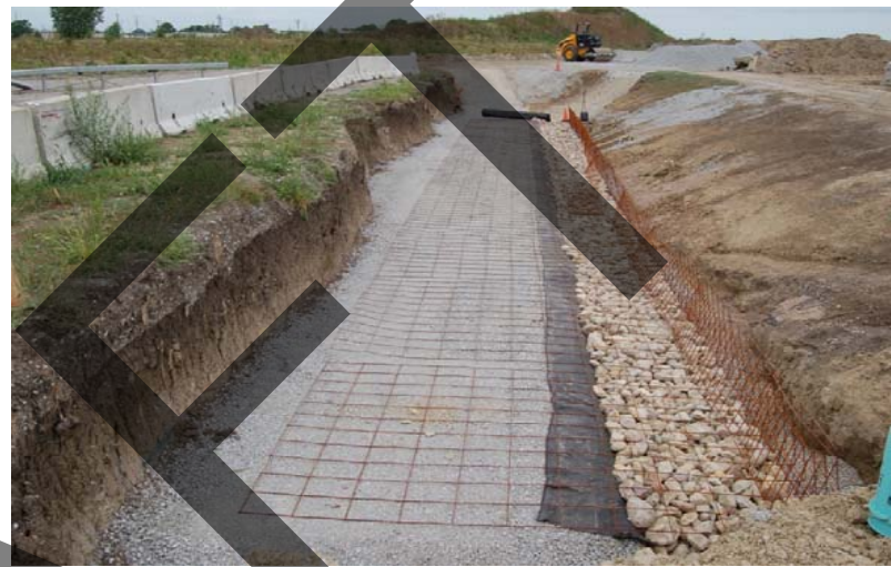
c. Wire Mat Final Allignment Before Filter Fabric
