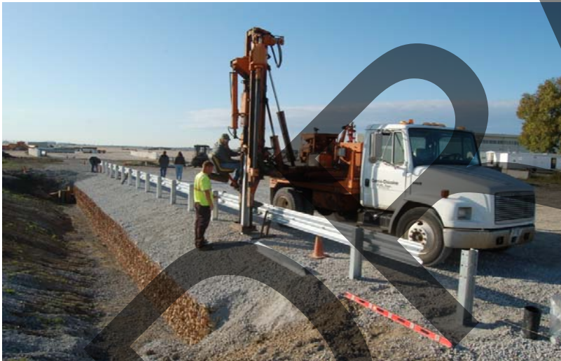
b. Non-Blocked MGS Installation, Driving Post No. 3
