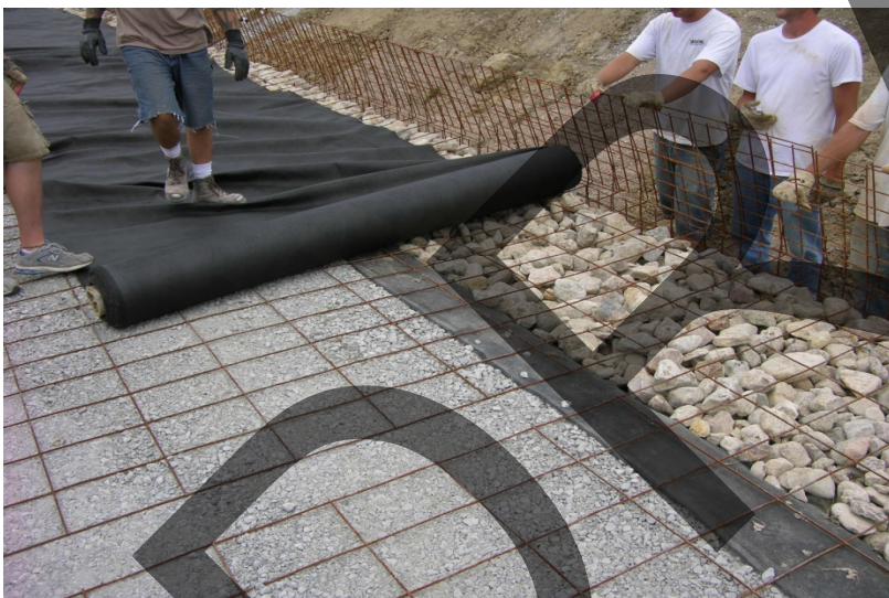
b. Rolling Out Fiber Filter
