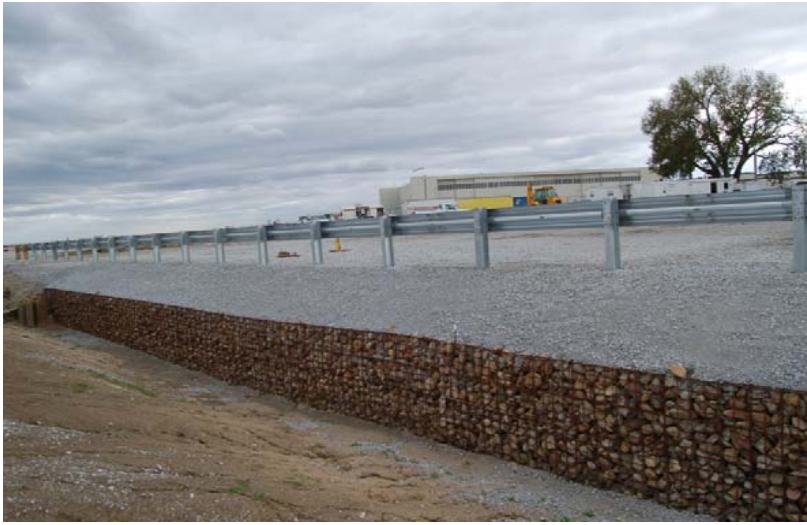
a. MGS on MSE Wall, Rear Quarter View
