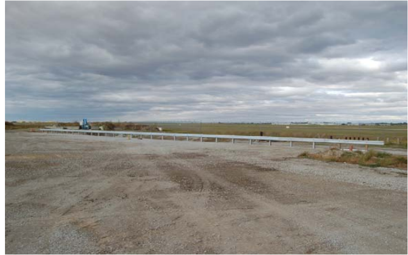
c. MGS on MSE Wall, Front View
