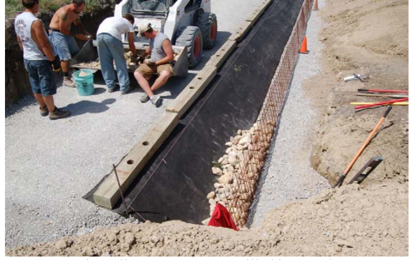
d. Wall Face Aggregate Filled by Hand
