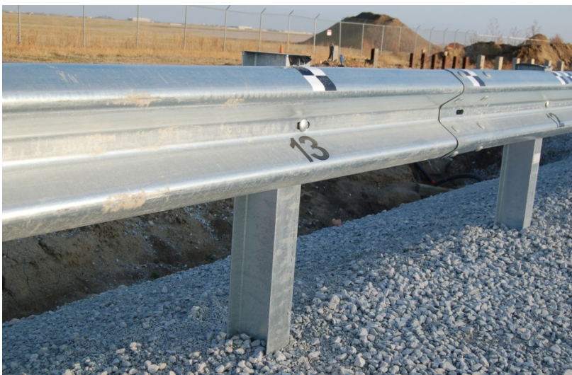
b. Downstream View of Post 13
