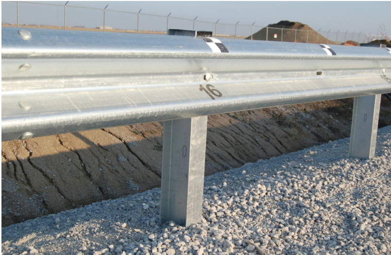
a. Downstream View of Post 16
