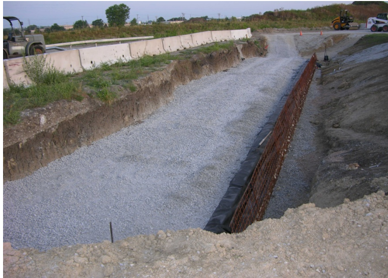
a. MSE Wall, Second Layer, Uncompact
