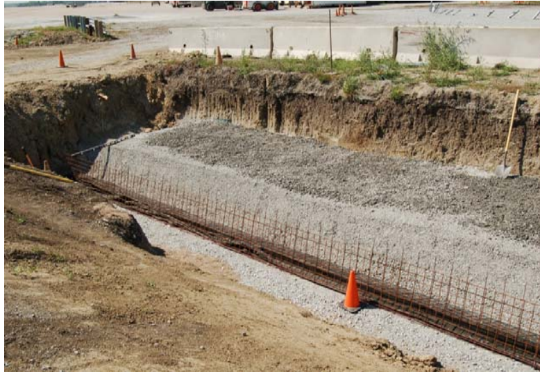
b. MSE Wall, First Fill Layer, Rear View
