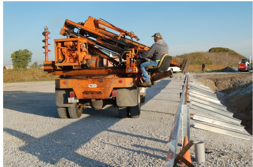
d. Non-Blocked MGS Installation, Driving Posts-1
