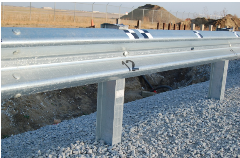
a. Downstream View of Post 12
