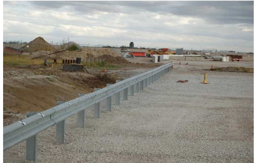
c. MGS on MSE Wall, Downstream Quarter View
