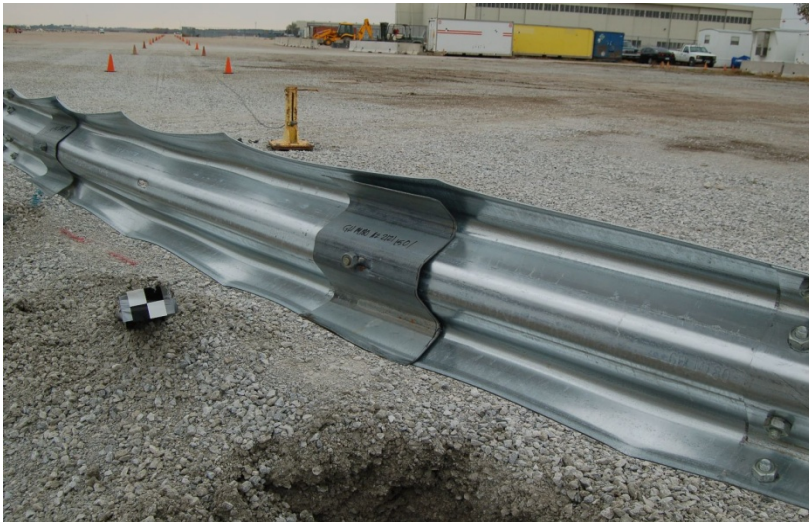
b. Rail at Post No. Back View
