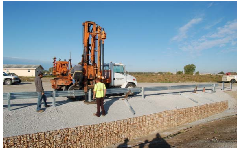
c. Non-Blocked MGS Installation, Driving Post No. 4
