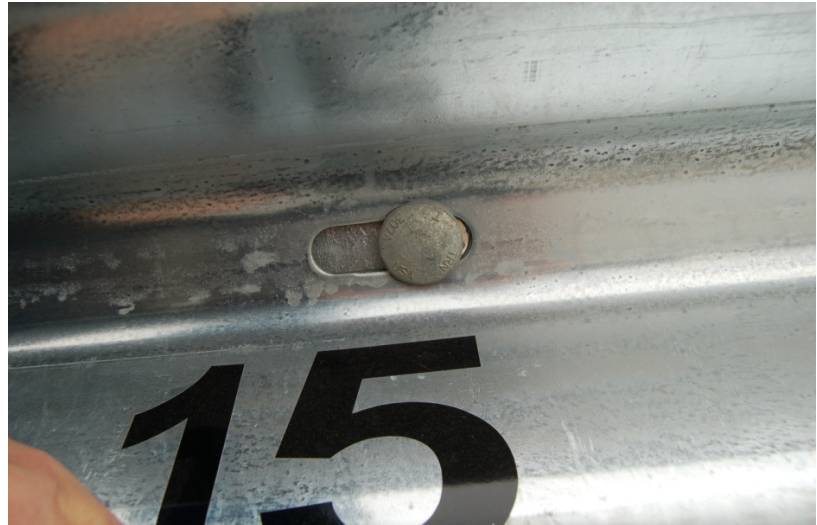
c. Bolt Location at Post 15
