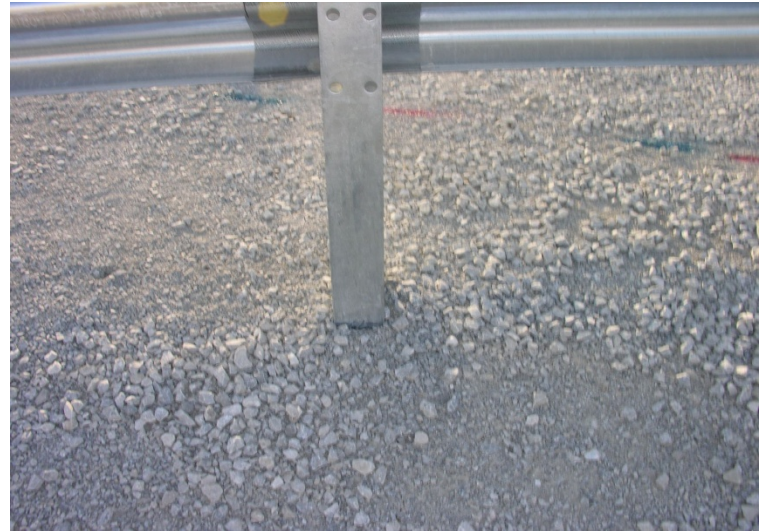
c. Post No. 11 Rear View
