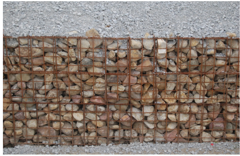
d. MSE Wall, Course Aggregate Close-up
