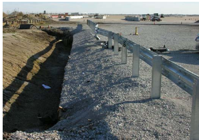
c. Downstream View
