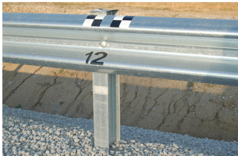
c. Upstream View of Post 12
