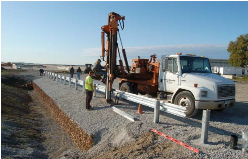
b. Non-Blocked MGS Installation, Driving Post No. 3
