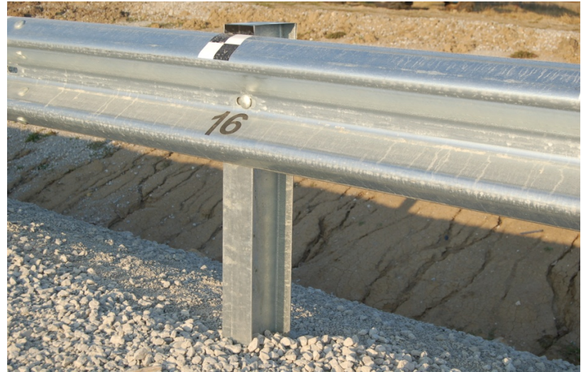
c. Upstream View of Post 16
