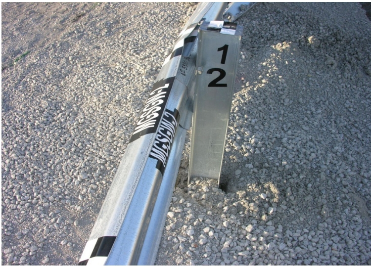
b. Post No. 12 Upstream View
