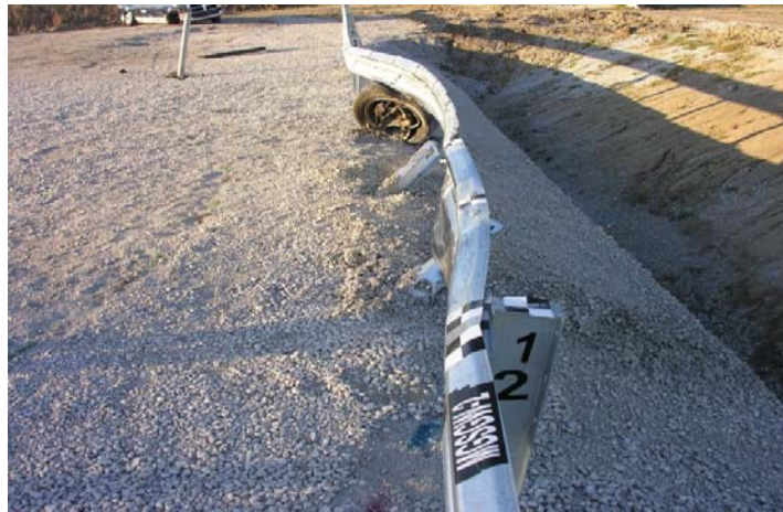
b. Upstream Inline View
