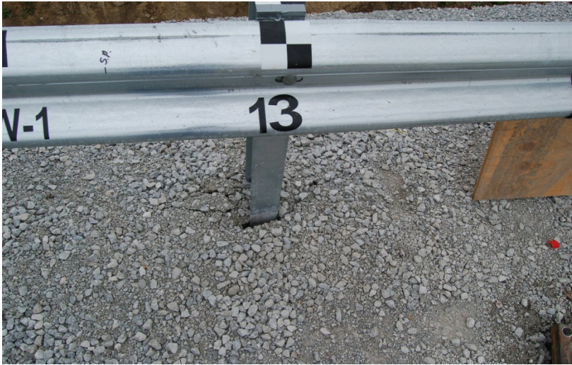
a. Post No. 13, Front Side
