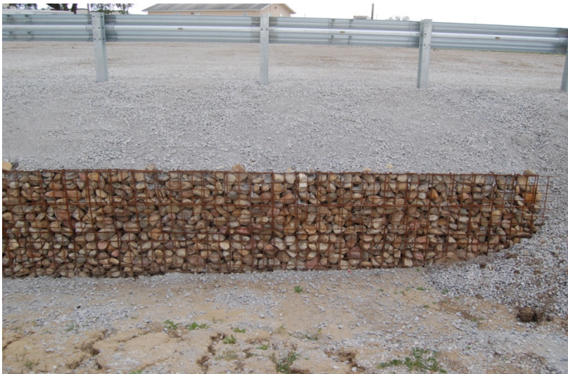
b. MSE Wall, Downstream End
