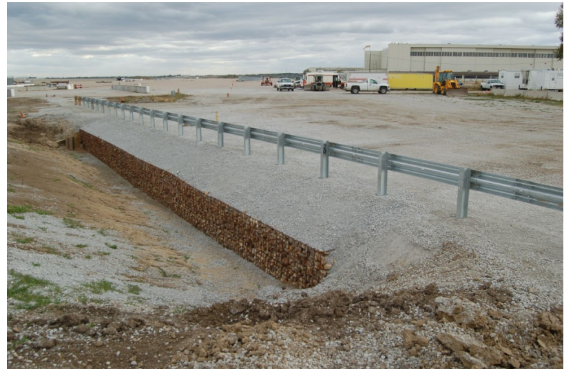
d. MGS on MSE Wall, Downstream Rear View
