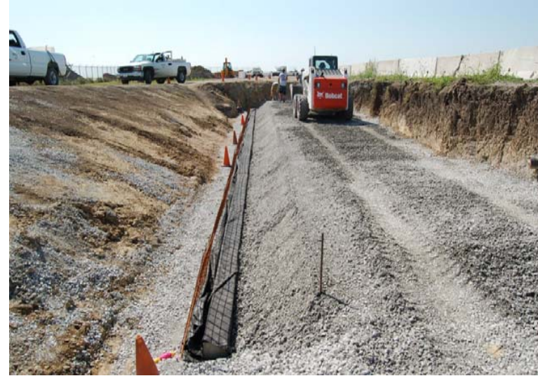
d. MSE Wall, First Fill Layer, Downstream View
