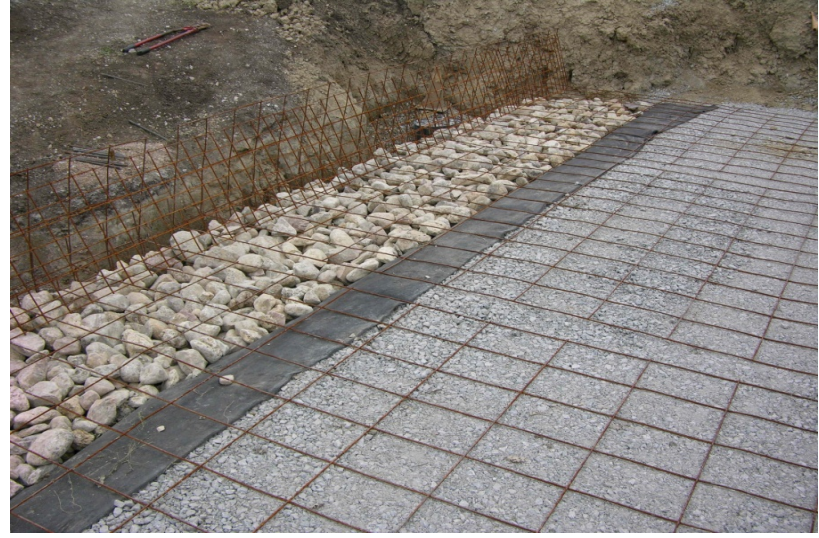
d. Second Layer Wire Mat Installed, Upstream End
