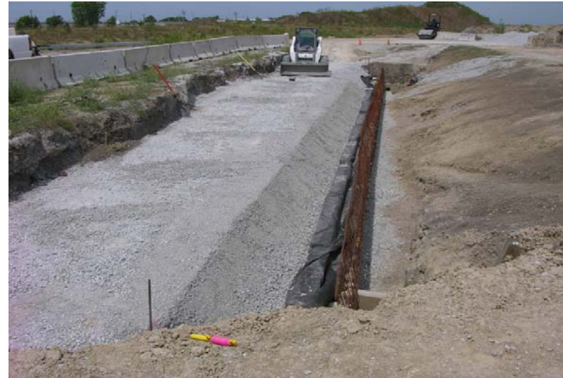
c. MSE Wall, Second Layer, Leveling
