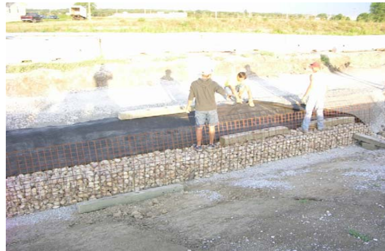
d. Second Layer Fiber Filter Positioning
