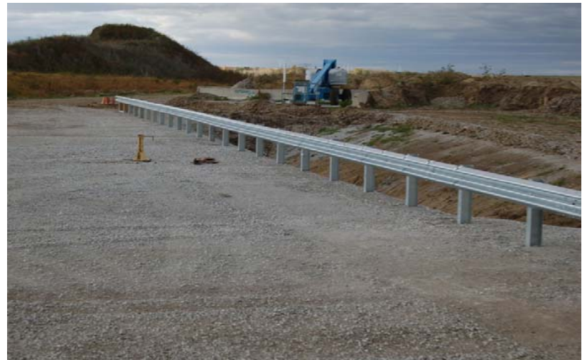
d. MGS on MSE Wall, Upstream Quarter View
