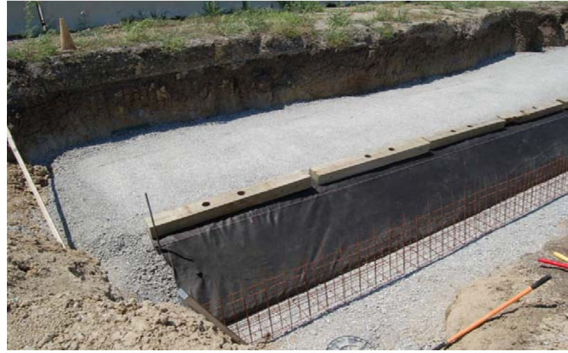
c. Filter Fabric Positioned
