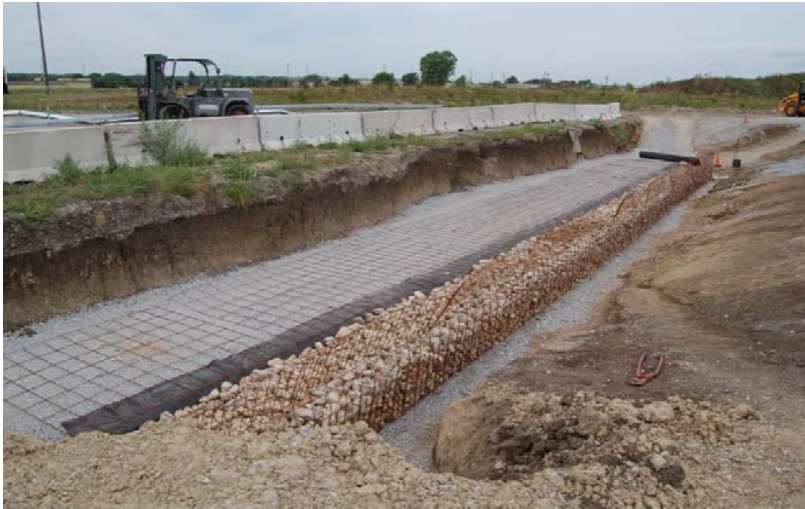
a. Second Layer Wire Mat Installed
