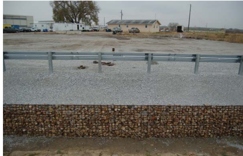
c. MSE Wall, Near Impact
