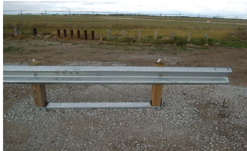
d. Front View of Upstream Anchor
