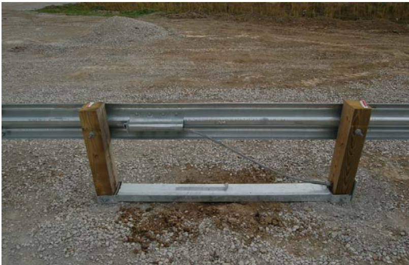
b. Rear View of Downstream Anchor
