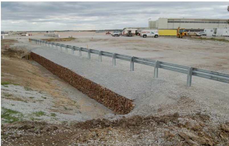
b. MGS on MSE Wall, Rear Quarter View
