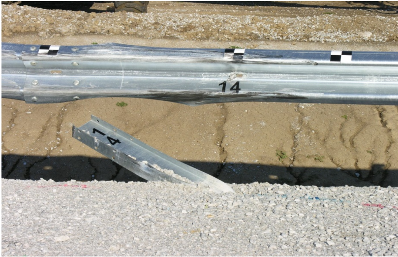
a. Rail at Post No. 14, Front View
