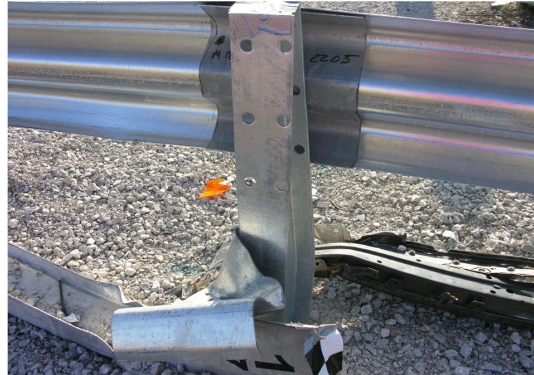
d. Post No. 18, Rear View
