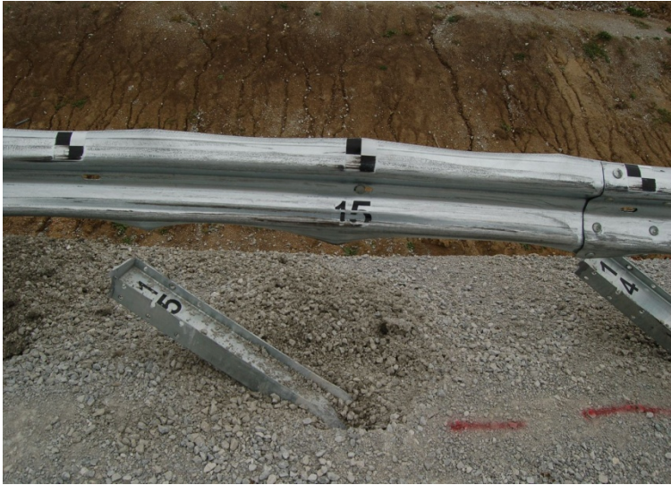
a. Post No. 15, Front View
