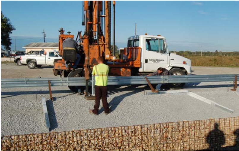
a. Non-Blocked MGS Installation, Driving Post No. 2
