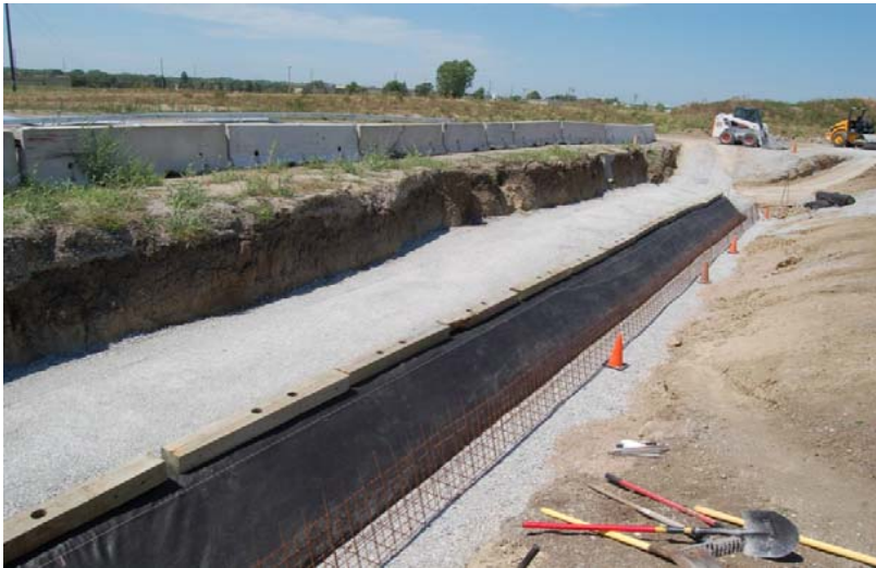
b. Fiber Filter Positioned, Ready for Course Aggregate
