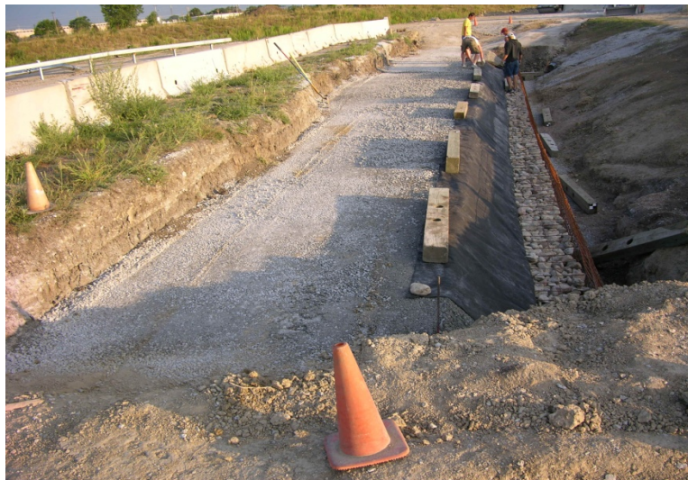
b. MSE Wall, Second Layer With Fiber Filter
