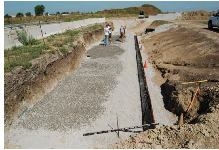
c. MSE Wall, First Fill Layer, Upstream View
