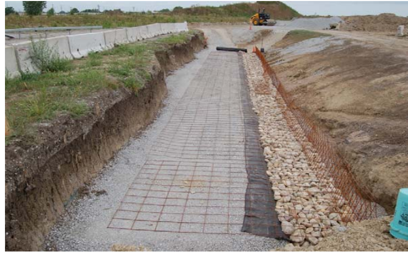
c. Wire Mat Final Allignment Before Filter Fabric
