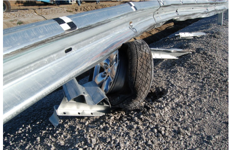
c. Post No. 15 Front View
