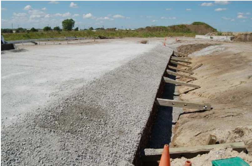
a. MSE Wall, Upstream View
