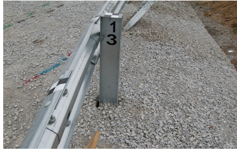
c. Post No. 13, Upstream View
