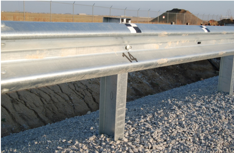
a. Downstream View of Post 14
