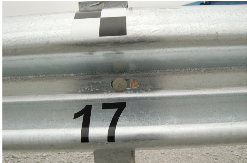
d. Bolt Location at Post 17
