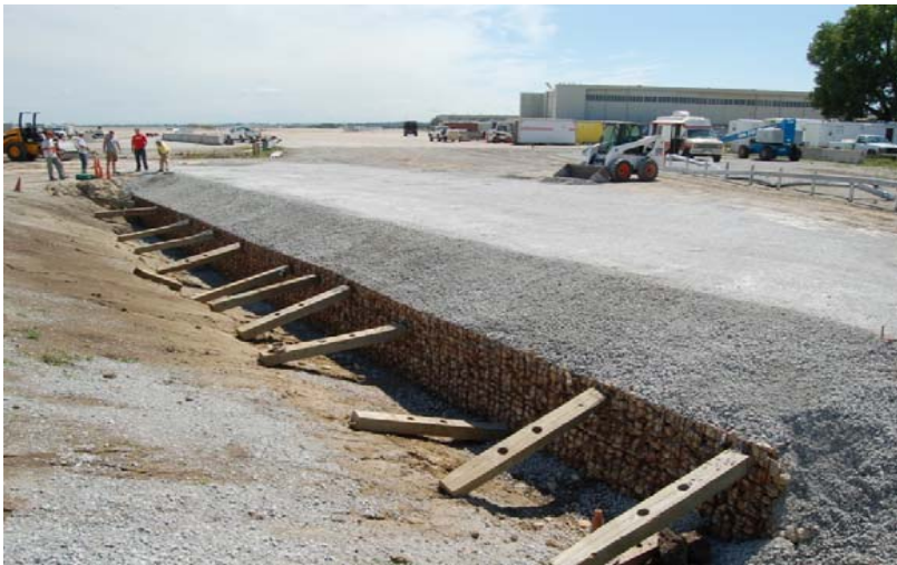
b. MSE Wall, Downstream View
