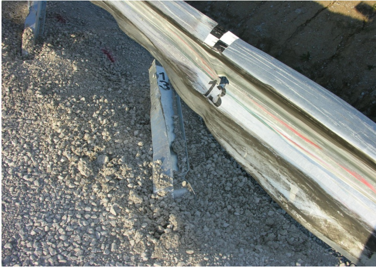
a. Post No. 13 Front View
