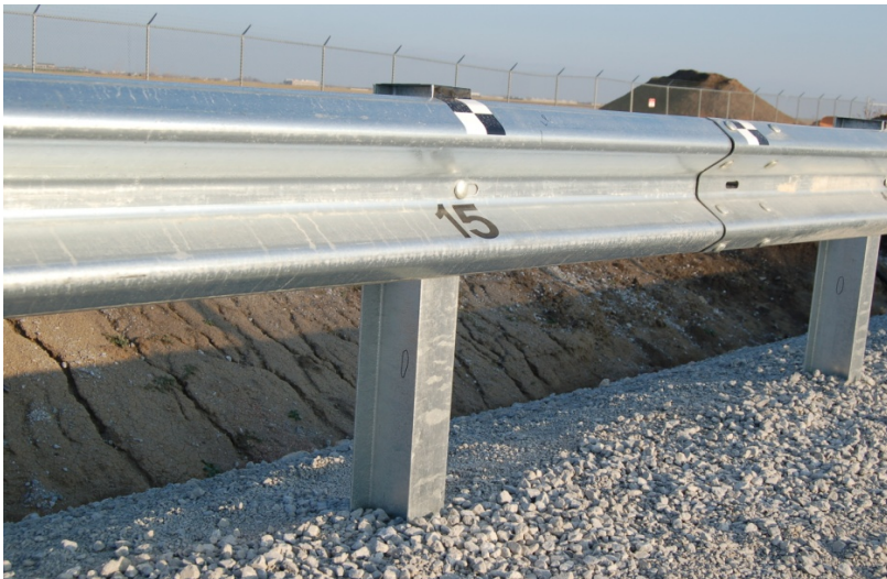
b. Downstream View of Post 15
