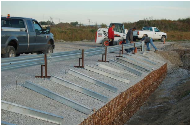
b. Non-Blocked MGS Installation, Leveling Rail
