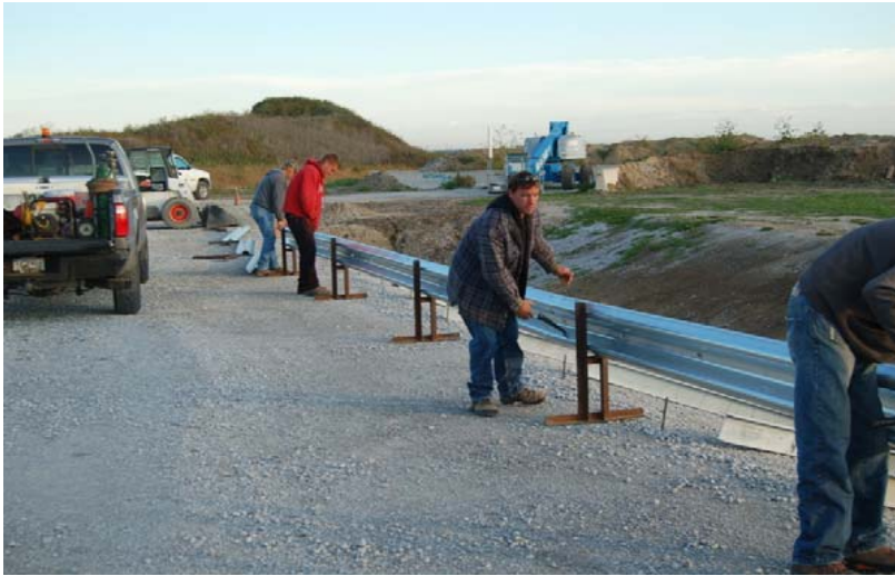
a. Non-Blocked MGS System Installation
