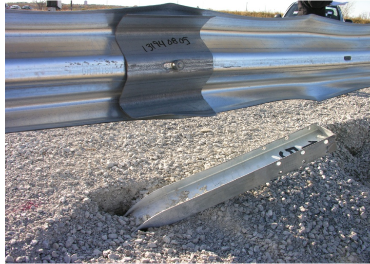
c. Post No. 15, Rear View
