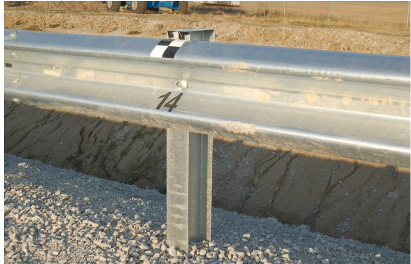
c. Upstream View of Post 14
