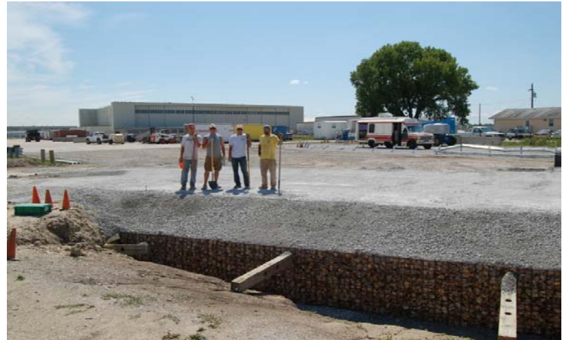
d. MSE Wall. Back View
