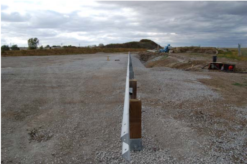
a. Upstream Inline View
