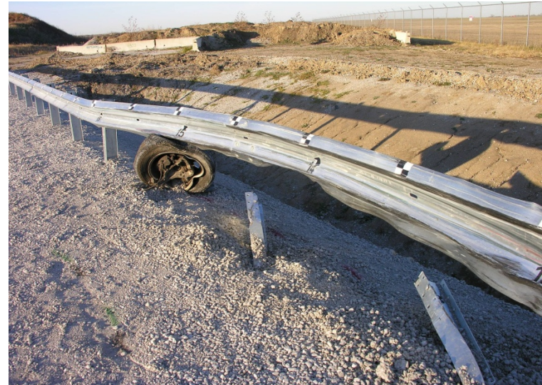
c. Impacted Rail, Front Quarter View
