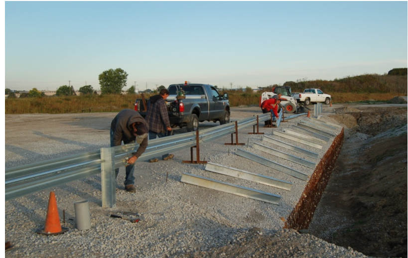
c. Non-Blocked MGS System, Initial Rail Attachment
