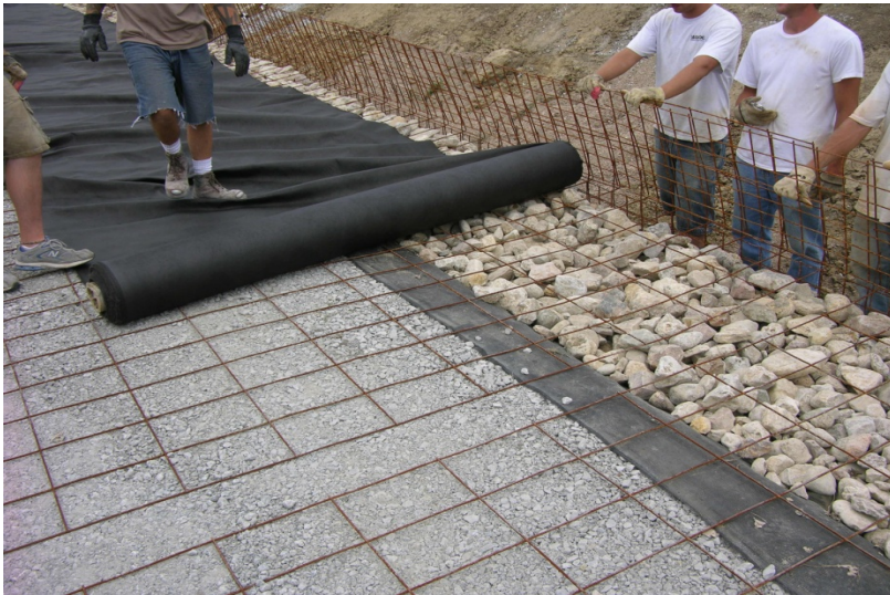
b. Rolling Out Fiber Filter
