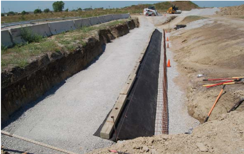
a. Filter Fabric Held by Posts
