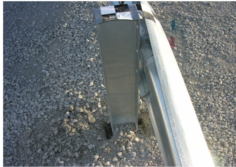
d. Post No. 12 Downstream View
