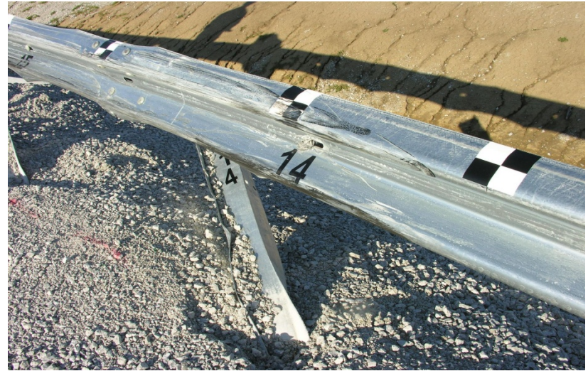
c. Rail at Post No. 14 Upstream Quarter View
