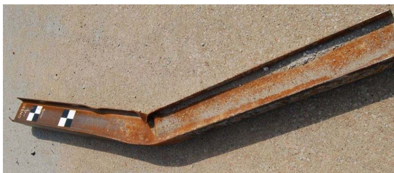
i. Post After Impact – Removed, Showing Deformation
