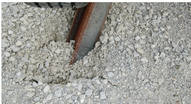
h. Post After Impact – Displaced Soil
