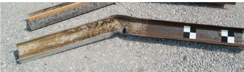
i. Post After Impact – Removed, Showing Deformation
