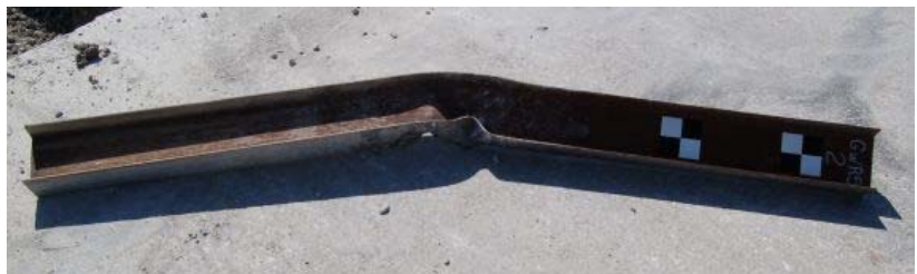
i. Post After Impact – Removed, Showing Deformation
