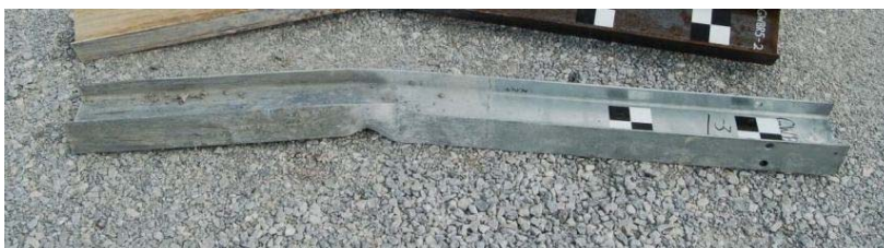
i. Post After Impact – Removed, Showing Deformation
