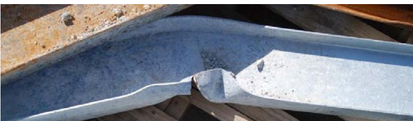
i. Post After Impact – Removed, Showing Deformation
