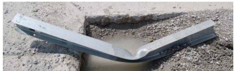
i. Post After Impact – Removed, Showing Deformation
