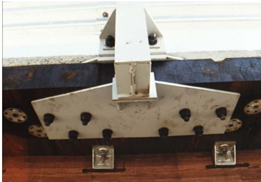
Figure 30. Steel Bridge Railing System - Bridge Posts
