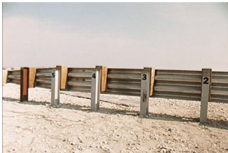
Figure 42. Approach Guardrail Transition - Back View
