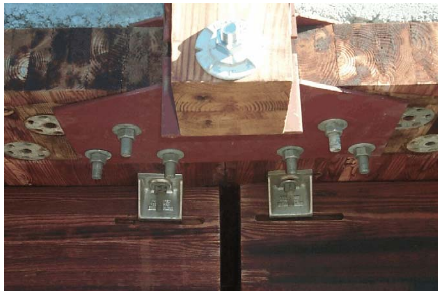
Figure 86. Wood Bridge Railing System - Bridge Posts
