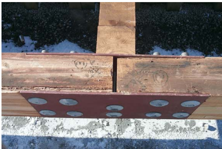
Figure 87. Wood Bridge Railing System - Rail Splices
