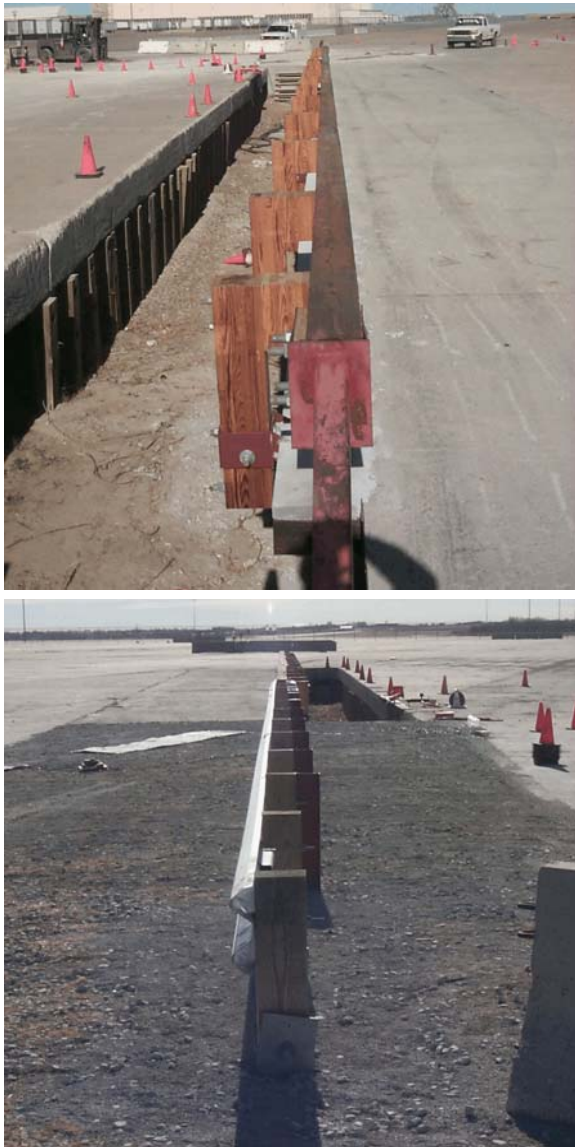
Figure 98. Approach Guardrail Transition - Parallel View
