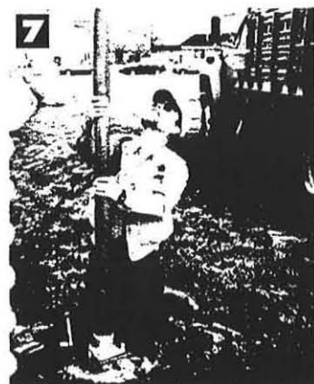
7 TURN POST AND POSITION SIGN IN PROPER DIRECTION.
