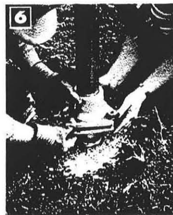
6 INSTALL BOLTS AND TIGHTEN NUTS LOOSELY.
