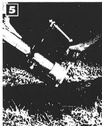
5 CLAMP E-Z LIFTING HINGE TO BASE STUB AND POST. LIFT INTO PLACE OVER BASE.
