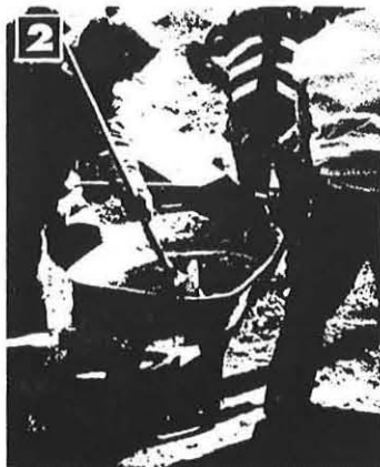
2 FILL HOLE TO GROUND LEVEL WITH CONCRETE.
