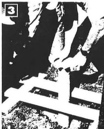
3 PRESS BASE INTO CENTER OF CONCRETE FILLED HOLE.
