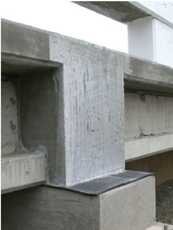
Figure 11. Lateral Stiffener End Caps at Bent Joints
