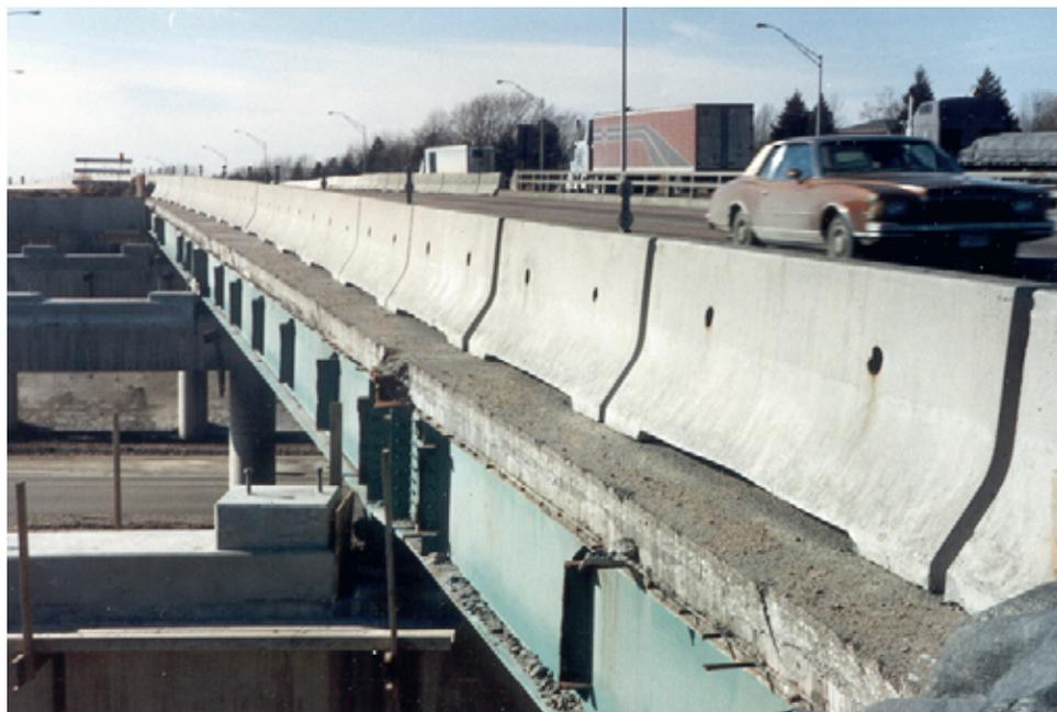
Figure 1. Temporary Barrier Positioned Near Bridge Deck Edge
