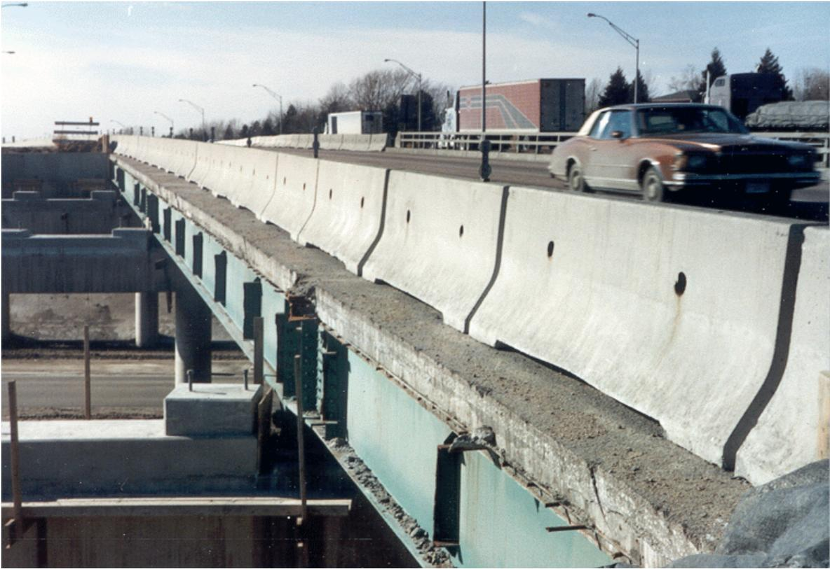
**Figure 1. Temporary Barrier Installation on Bridge Deck**
