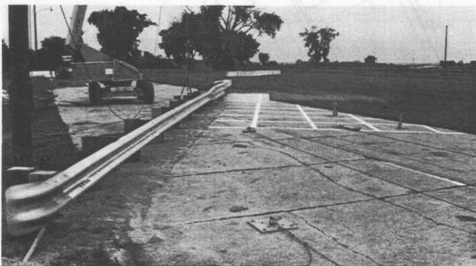
Figure 9 PHOTOGRAPHS OF APPROACH GUARDRAIL INSTALLATION
