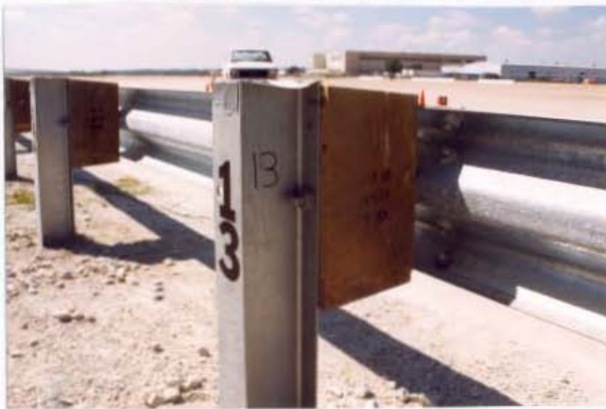
Figure 4. Post-to-Rail Attachment for the Type B (W-beam) Longitudinal Barrier System
