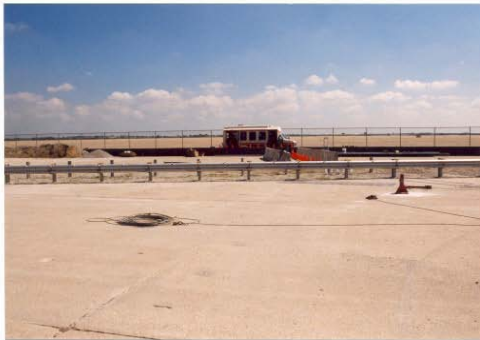
Figure 2. Type B (W-beam) Longitudinal Barrier System
