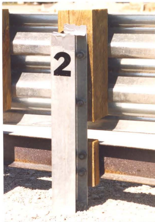
Figure 8. Approach Guardrail Transition, Design No. 1 (Continued)
