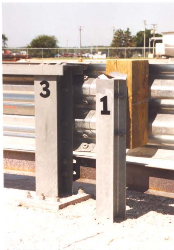
Figure 8. Approach Guardrail Transition, Design No. 1 (Continued)
