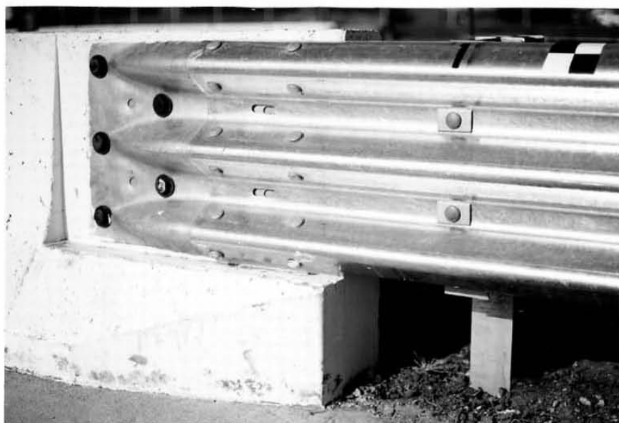
Figure 4. Modified Bridge Anchor Section
