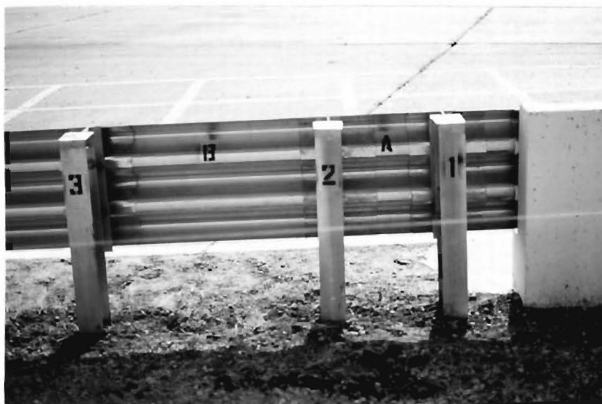
Figure 5. Modified Bridge Anchor Section
