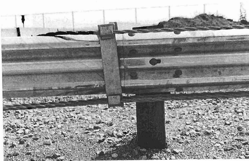
Figure 5. Transition Cable Brackets.
