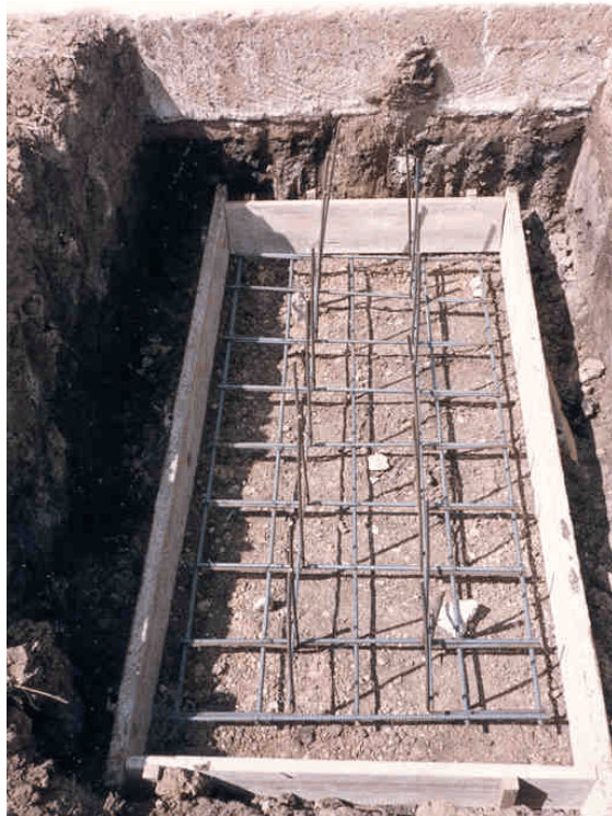
Figure 2. Construction of Concrete Bridge Supports.
