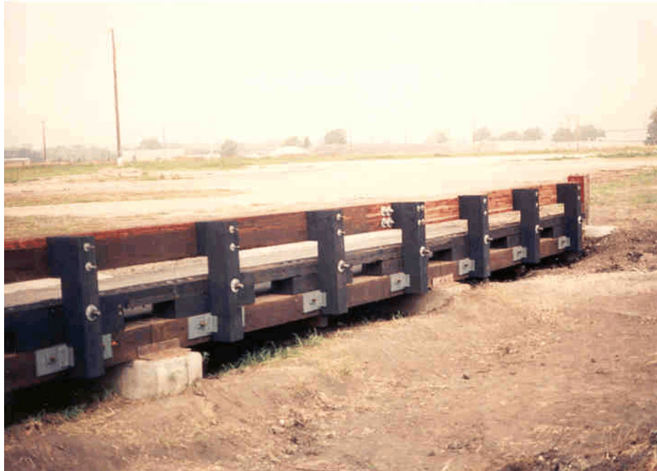
Figure 24. Bridge Railing System - Bridge Posts
